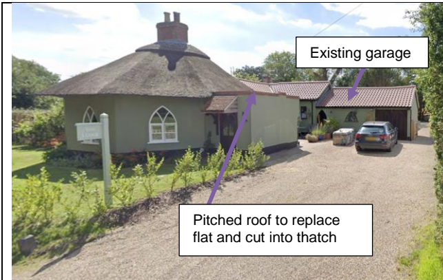
Front of property showing the thatched roundel and existing garage (to be demolished) and parking.
