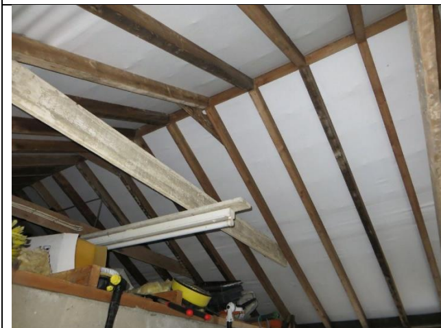
Inside existing garage. New roofing membrane under tiles. No evidence of current or of previous use by bats.
