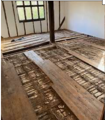
Boxing, hiding the RSJ beneath
