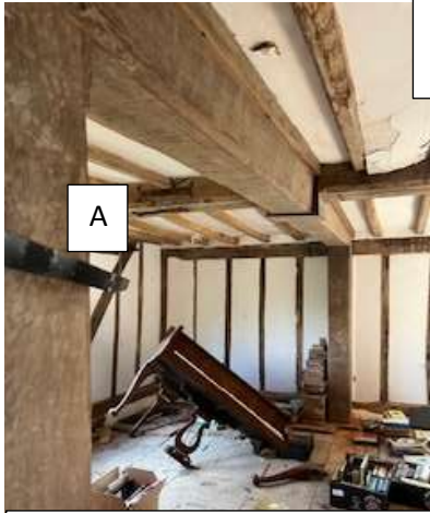
Boxing, hiding the RSJ beneath
