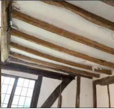
Whilst most timbers appear sound, the most easterly bay shows as many as 5 badly deteriorated floor joists. One is visibly broken through.
