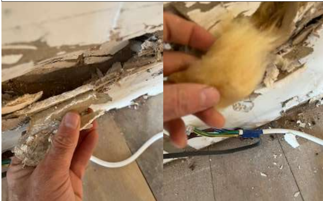
Large bathroom to be divided in two. Modern plasterboard seen. Modern timbers to stud work. Fibre glass insulation.
