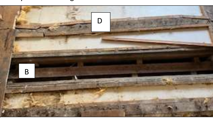
RSJ replacement of original timber
