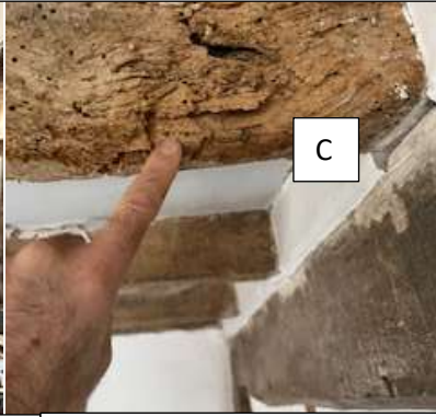
Whilst most timbers appear sound, the most easterly bay shows as many as 5 badly deteriorated floor joists. One is visibly broken through.
