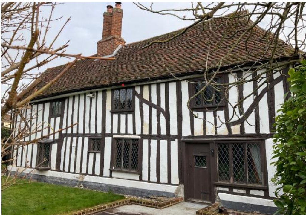
Picture 8: West Elevation
