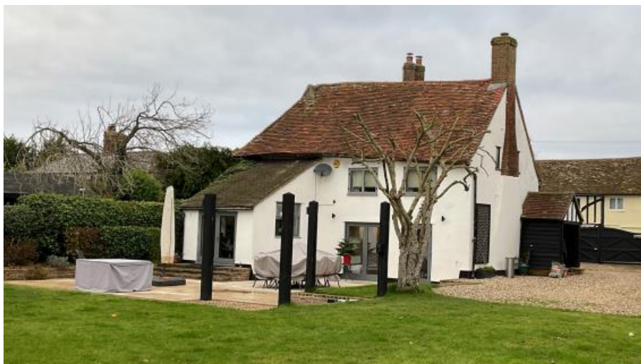
Picture 9: South East Elevation
