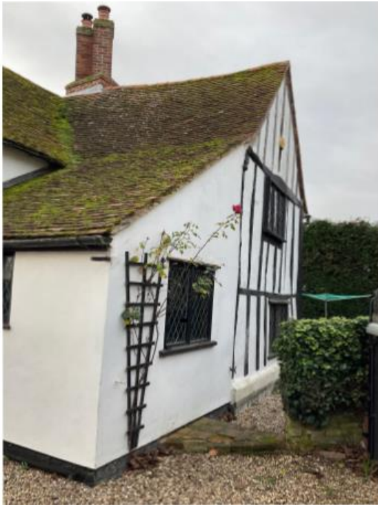
Picture 7: North Elevation
