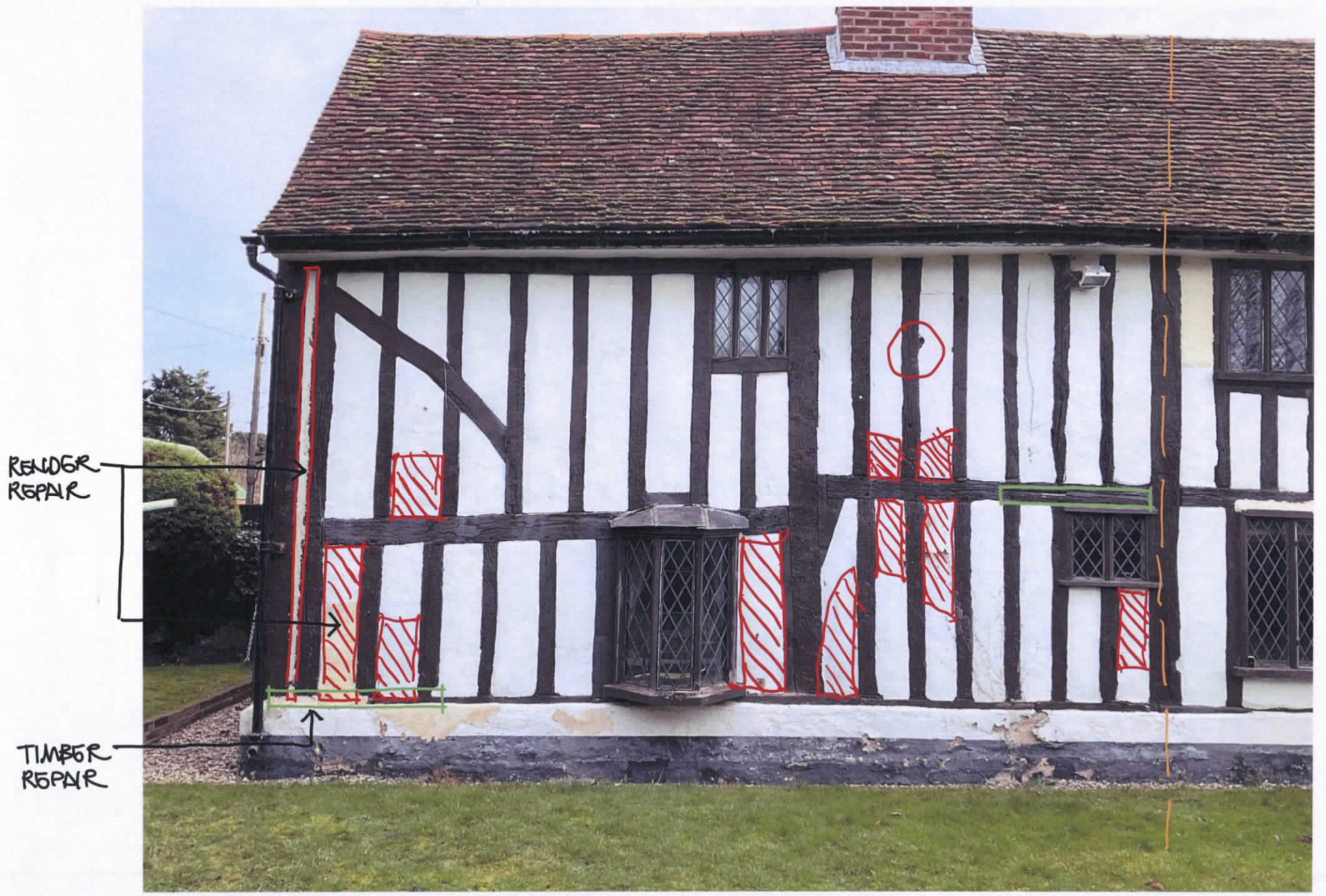
WEST ELEVATION - NORTH END - RENDER AND TIMBER REPAIRS
