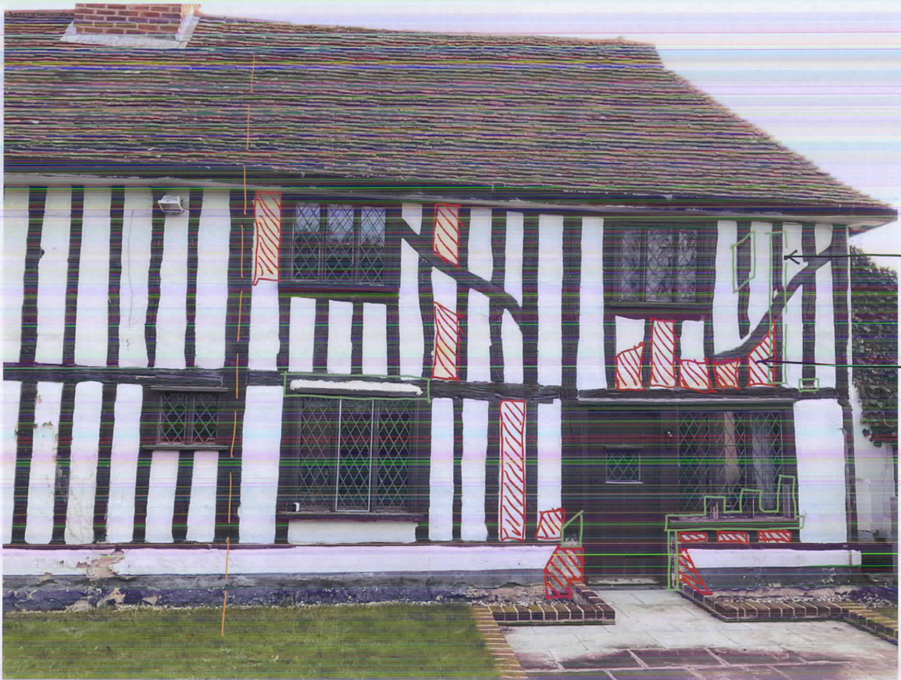
WEST ELEVATION - SOUTH END . RENDER AND TIMBER REPAIRS .
