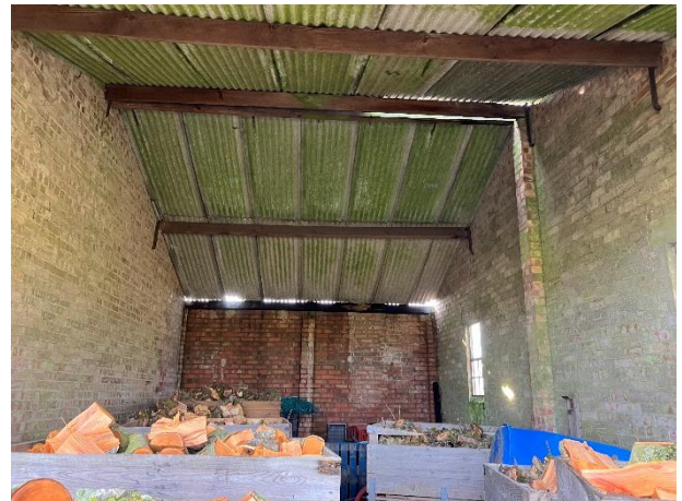
Photo 8: Internal view of western building bay
