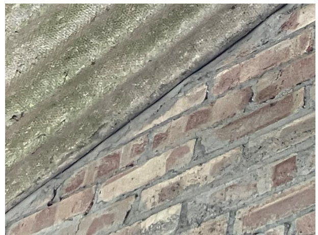
Photo 10: Roof sheets well cemented to top of brick wall
