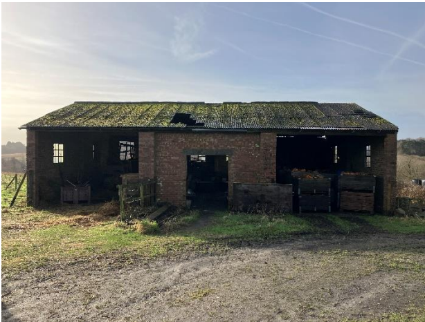
Photo 1: Northern façade of building
