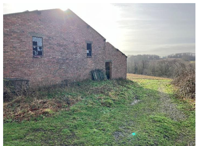
Photo 4: Western façade of building, with adjacent track leading south
