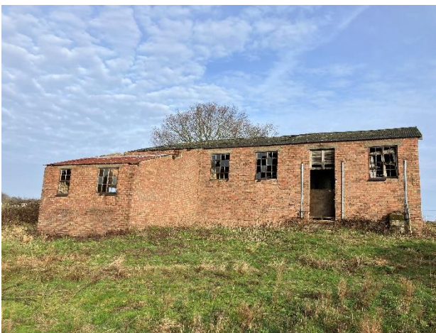
Photo 3: Southern façade of building, with grassland extending away to south
