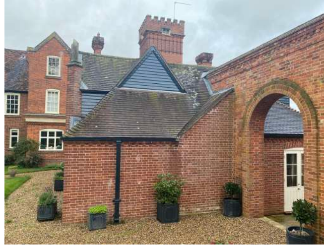
2. Materiality of Grade II Listed Nether Hall.
