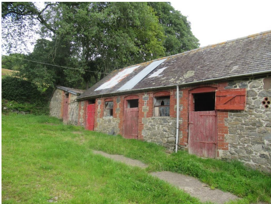
Figure 4.3. External view of the northern side of the barn
