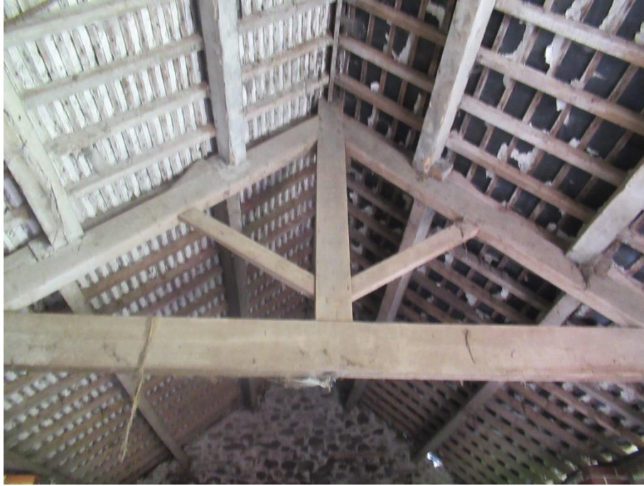
Figure 4.6. Roof space of middle section
