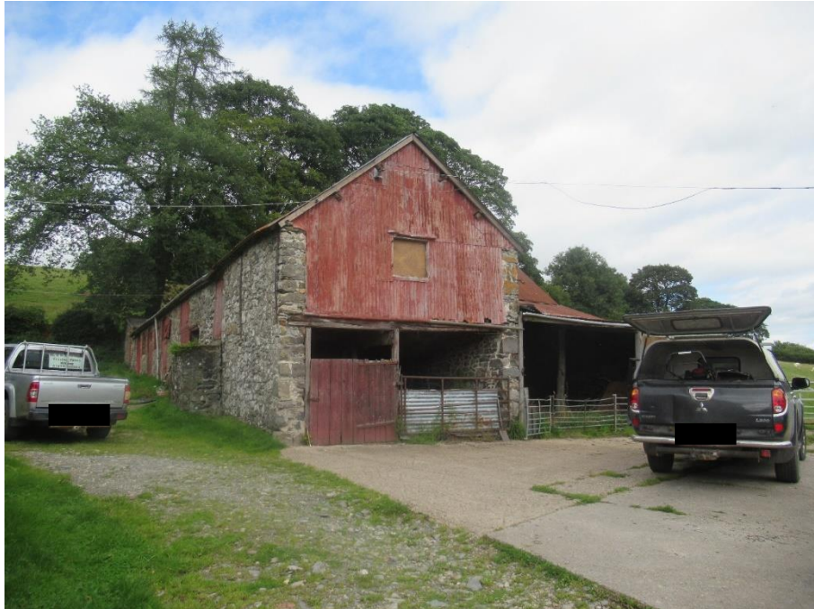
Figure 4.2. External view of the barn from the southwest
