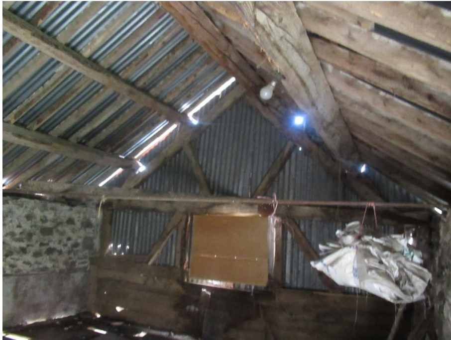
Figure 4.7. Southwest room on upper floor
