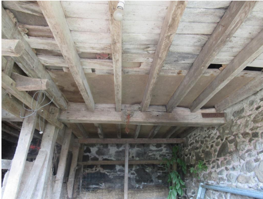
Figure 4.4. Ground floor of southwest corner
