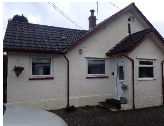
Figure 3. The west elevation of the property
