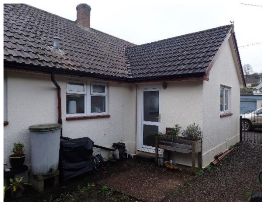
Figure 5. The property viewed from the northeast
