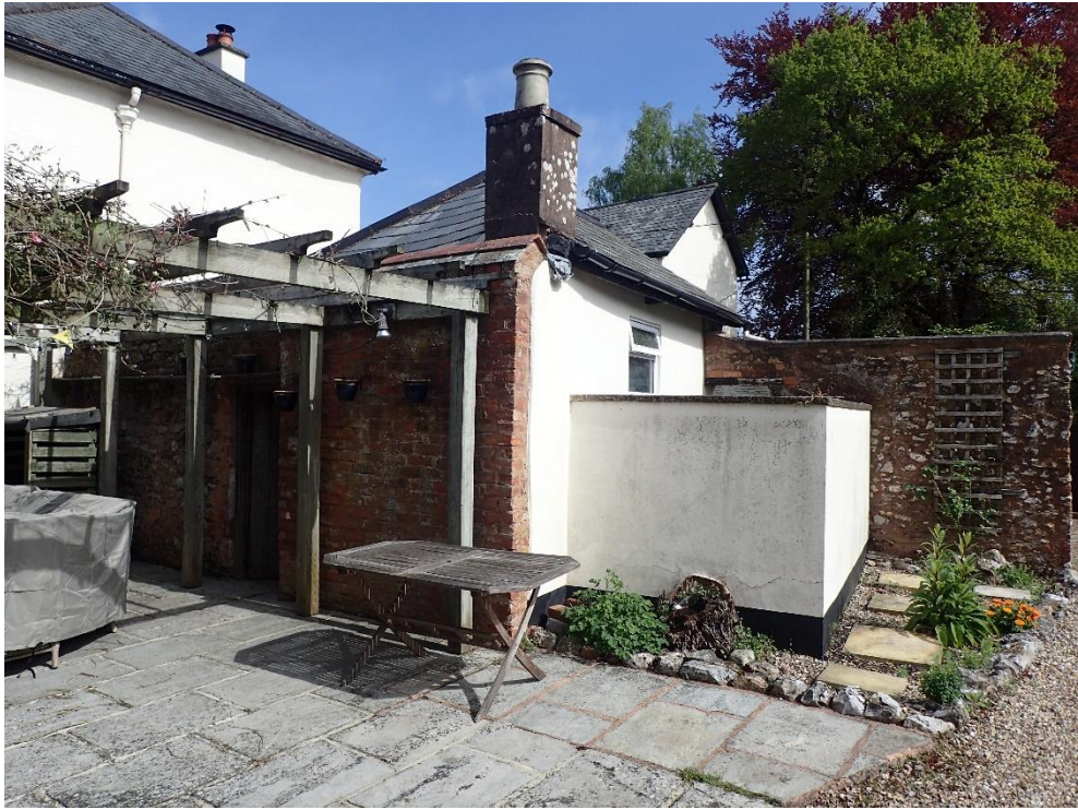
Figure. 3 The rear of the former coach house viewed from the south
