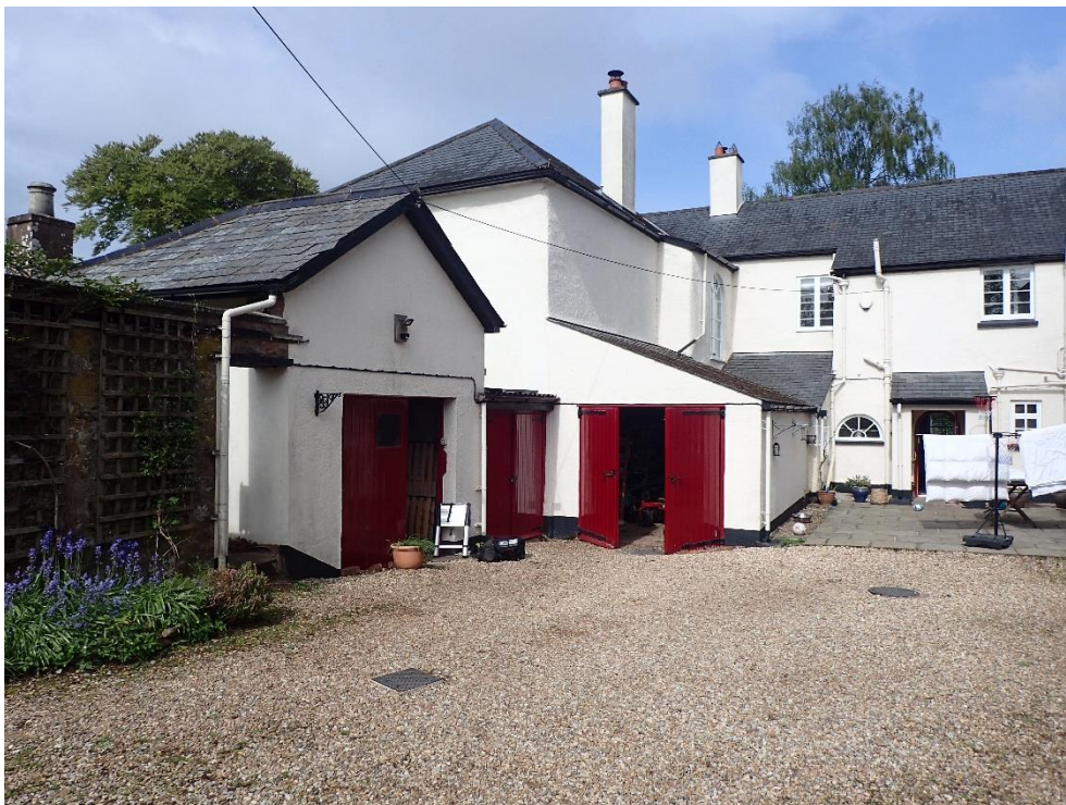
Figure. 2 The single storey extension to the house and former coach house viewed from the east
