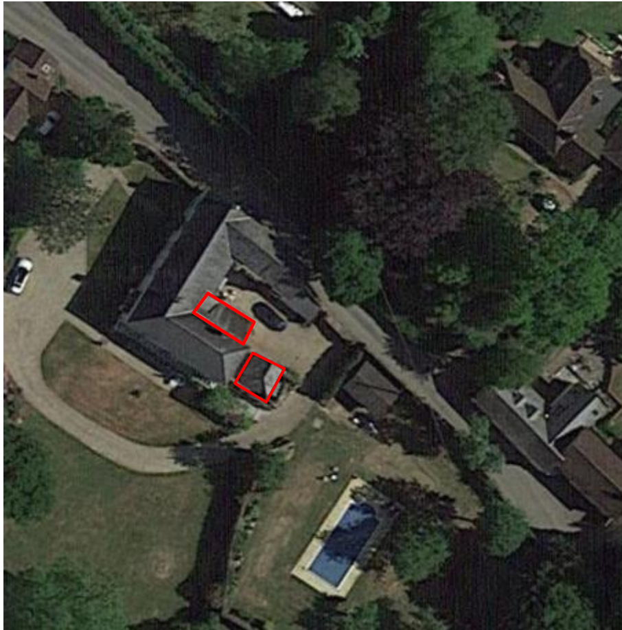
Figure. 1 Plan view of Craddock Lodge with rear extensions and coach house highlighted in red.
