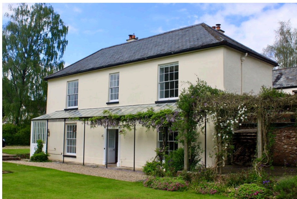
View of the south facing Georgian wing. This will be unaffected by the proposals.
