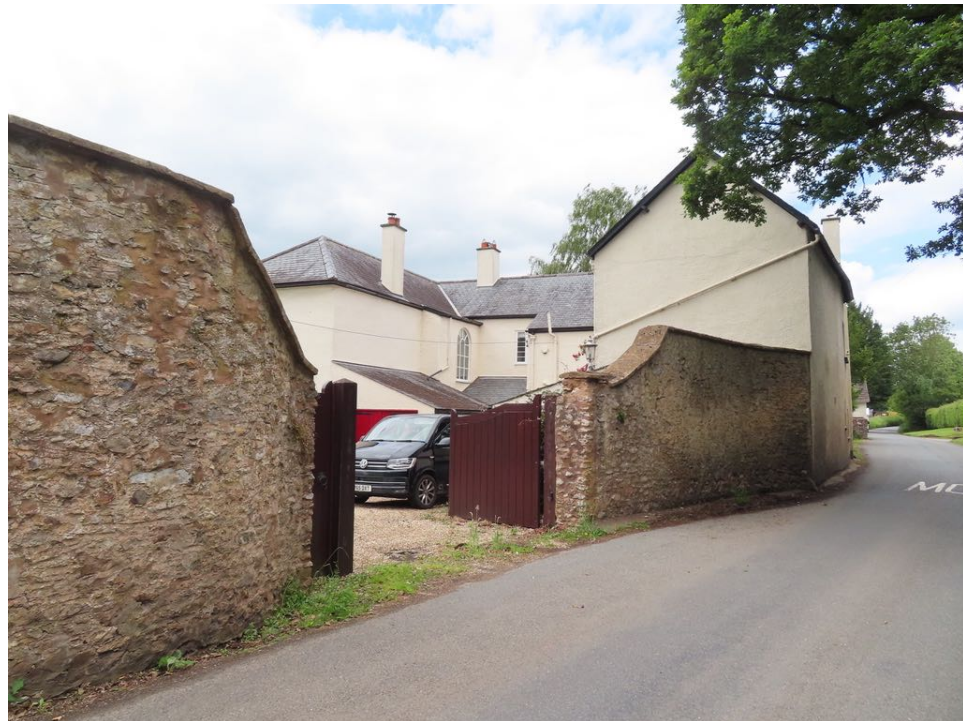
Photo of the northern facade addressing the public road. The original coach house and stables entrance. Gable end wall of the main house. The proposal being to continue the exposed stone as a plinth at street level with lime render above.
