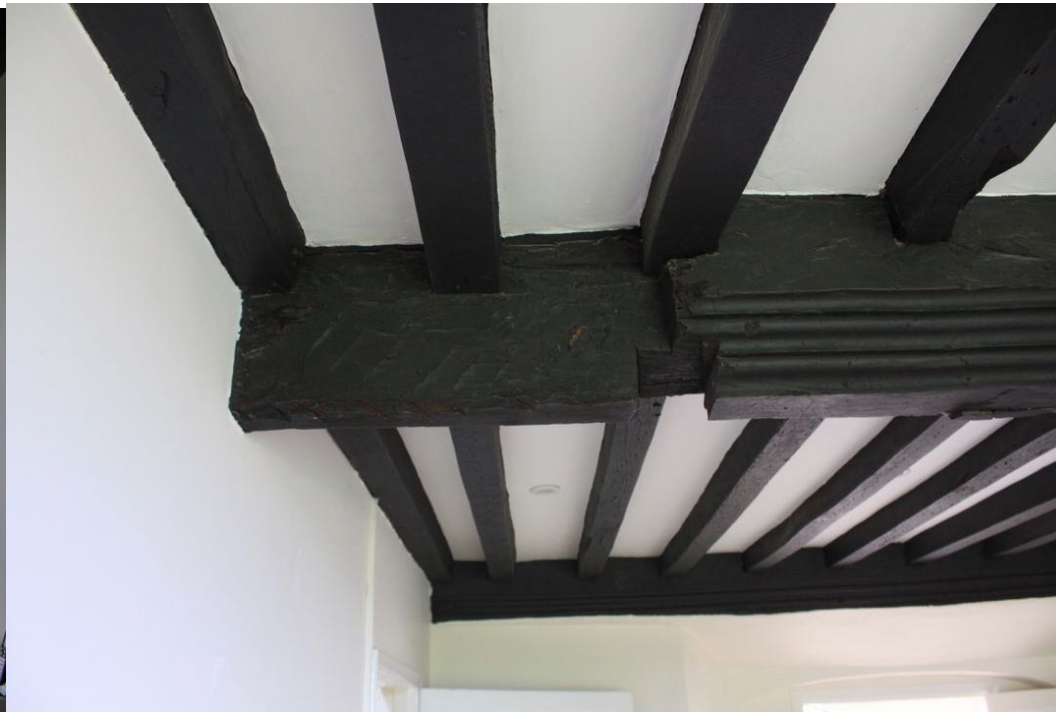
The beams as original elements remain largely intact, the ends have been modified. Ornate moulding on the main ceiling beams.
