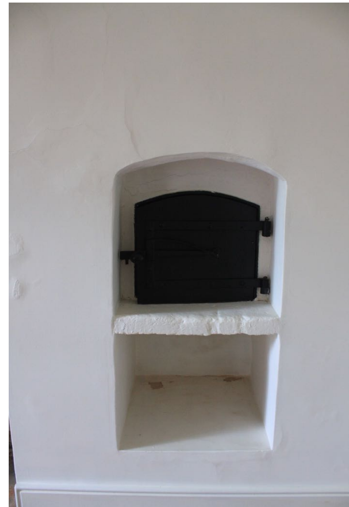
View of the bread oven located in the north western corner main room form the original Devon longhouse.
