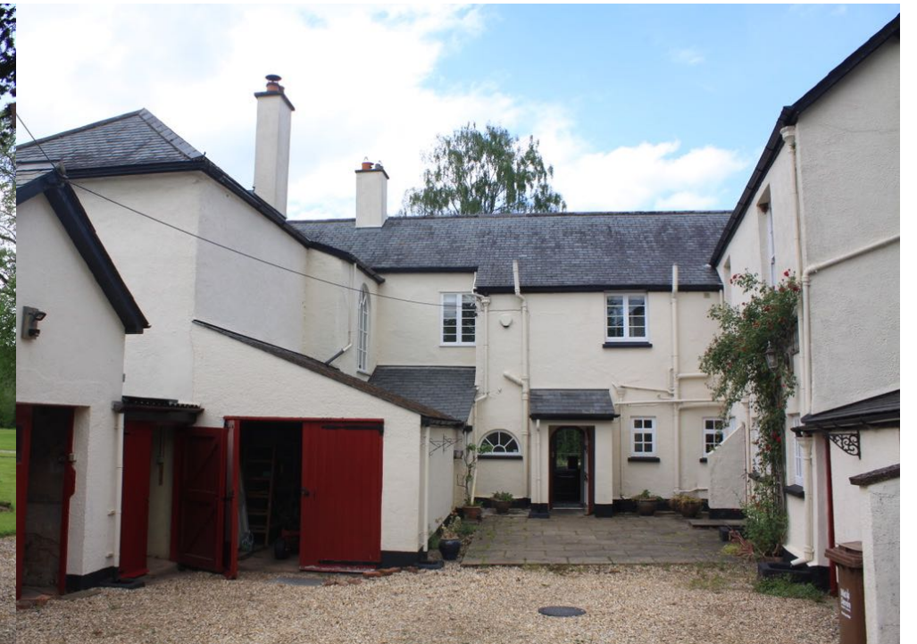
Photo of the courtyard showing the typically piecemeal evolution of this type of back of house area. The proposed window replacements are around this courtyard.
