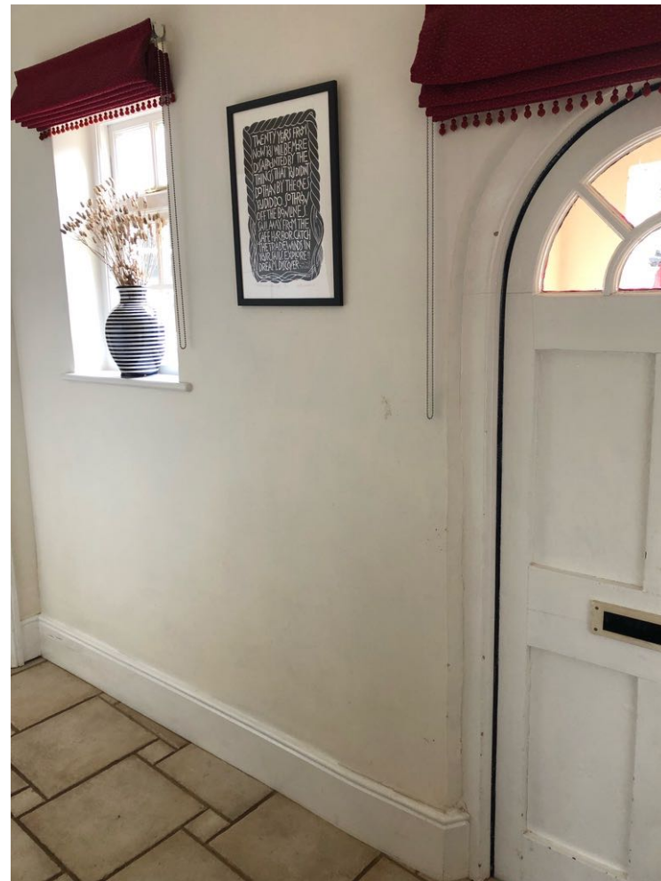
The 19th C corridor showing different window types, the early 20th C porch and modern door. These will be removed with the solid wall areas retained.
