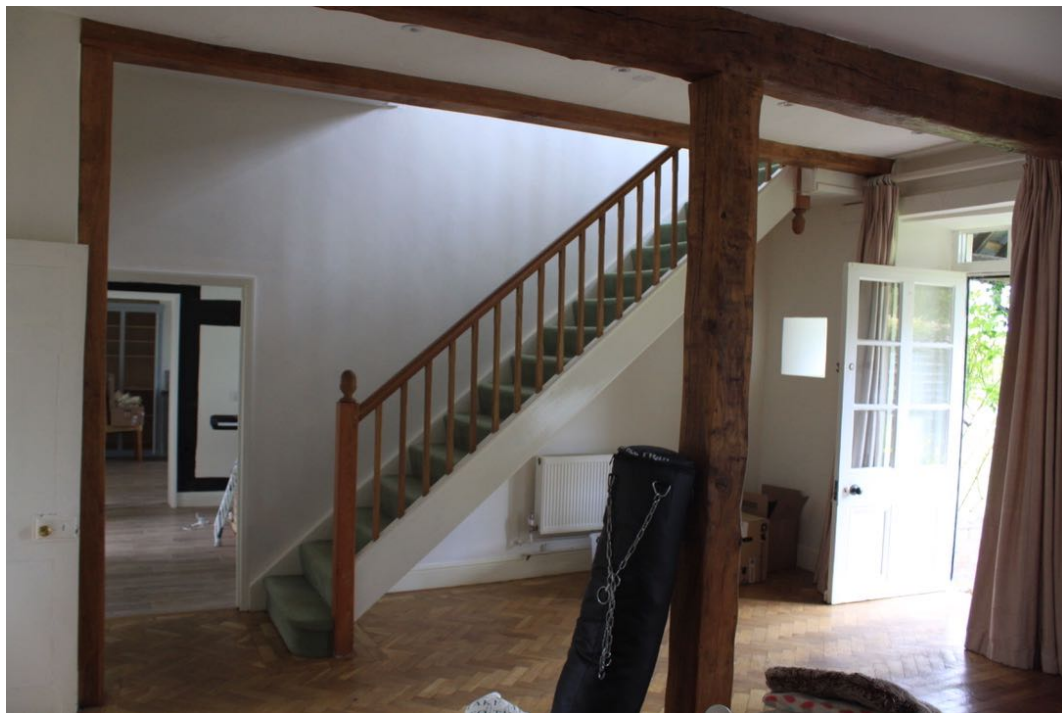
The secondary 20th C stair and opened up internal wall. The proposal is to swap the flight of this stair for more efficient circulation up at first floor and be less intrusive at ground floor.
