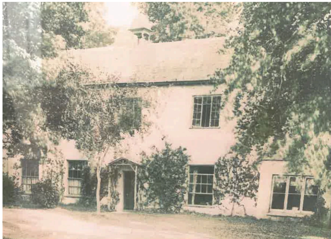
Photograph circa 1900. West facing facade. Showing the original entrance door location and sash window arrangement. Existing first floor windows are 20th C replacements now.
