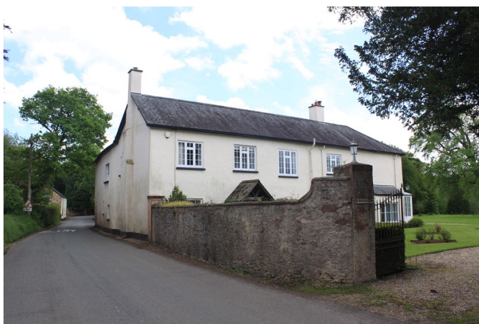
View from the public lane and the vehicular entrance on the north western side. The existing stone boundary wall will continue as a plinth at street level along the building.
