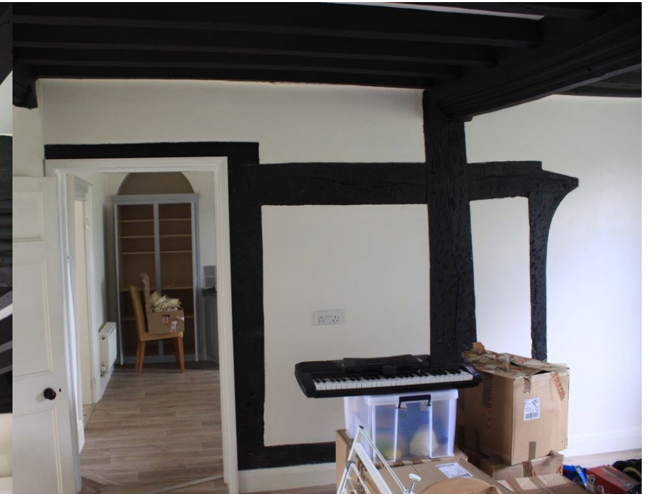
View looking down the original long house.
