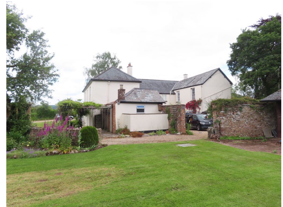
Photo of the eastern facade - the coach house, courtyard and outbuilding side. Secondary vehicle entrance, former stables and outbuildings with access to the gardens. The roof on the right hand side will be replaced with natural slate.
