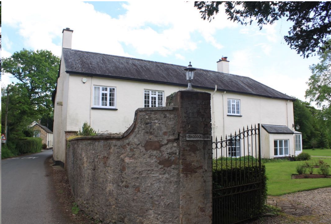
Photo of the northern and western facades from the public road.
