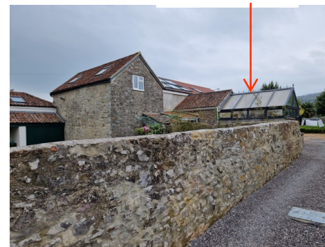
boundary wall to the Laurels
