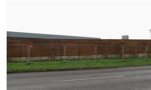
Existing view of the east elevation from the A1101.
