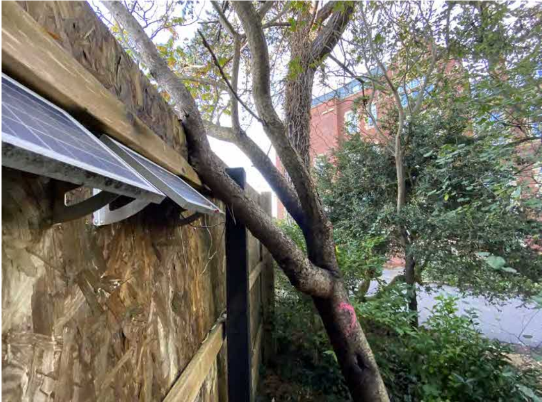
Photographic plate showing T41444, dead and leaning north damaging fencing and overhanging public footpath. (ROAVR, 2023)
