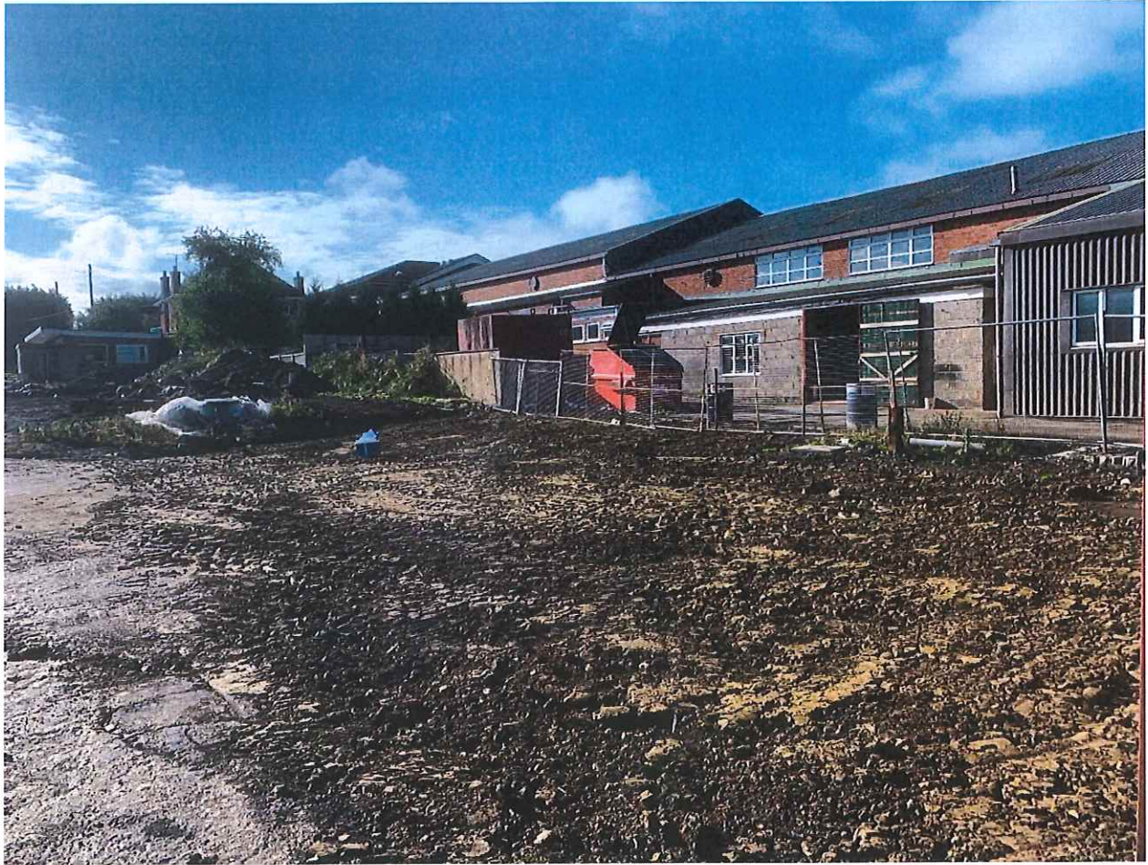
View of backfilled Excavation Looking South
