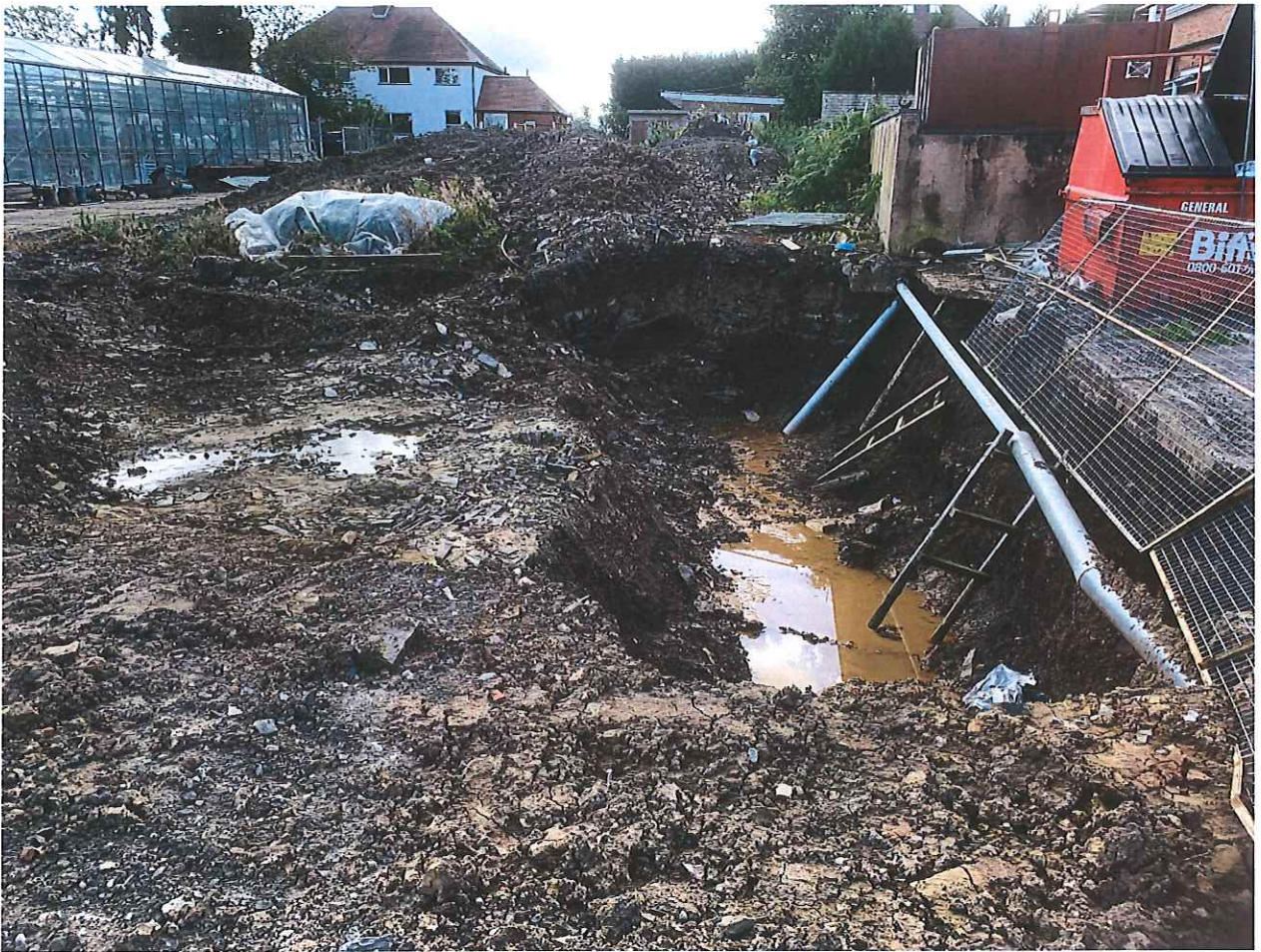
Extent of Excavation Looking South
