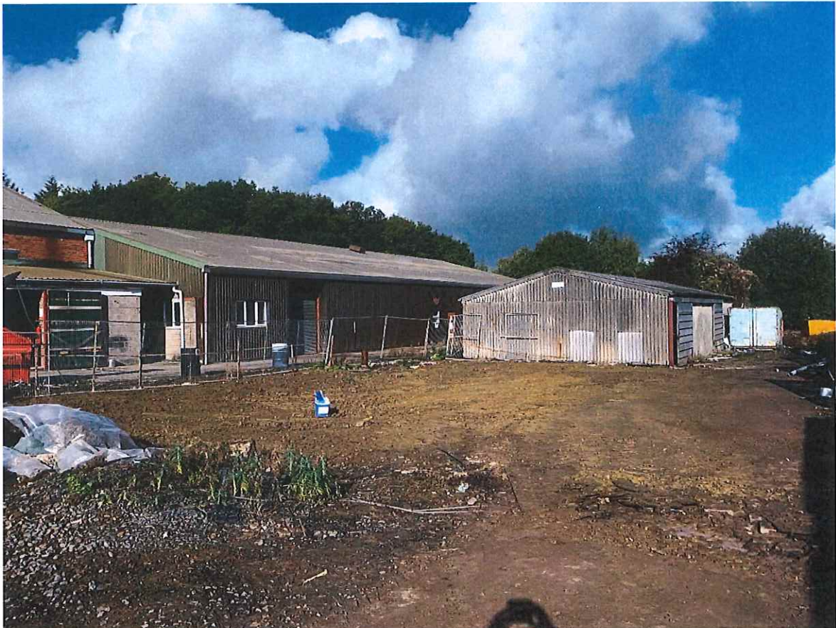
View of Backfilled Excavation Looking North
