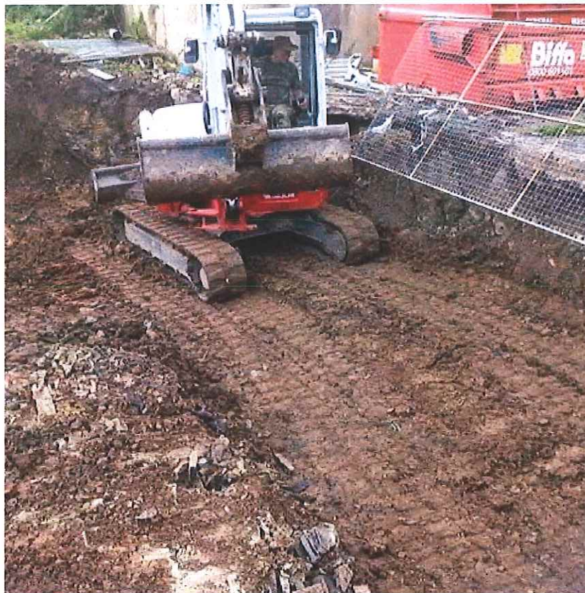
Excavation Being Backfilled with Clean Clay
