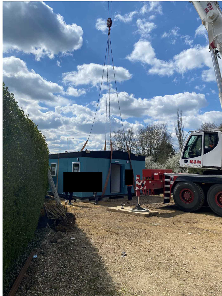
Installation of temporary portable cabin took place in April 2021.
