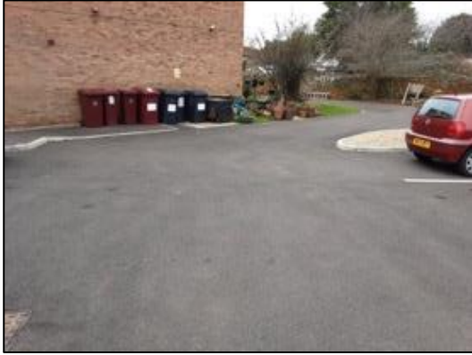
Photograph 1. The northern boundary car park, leading to the site's entrance.
