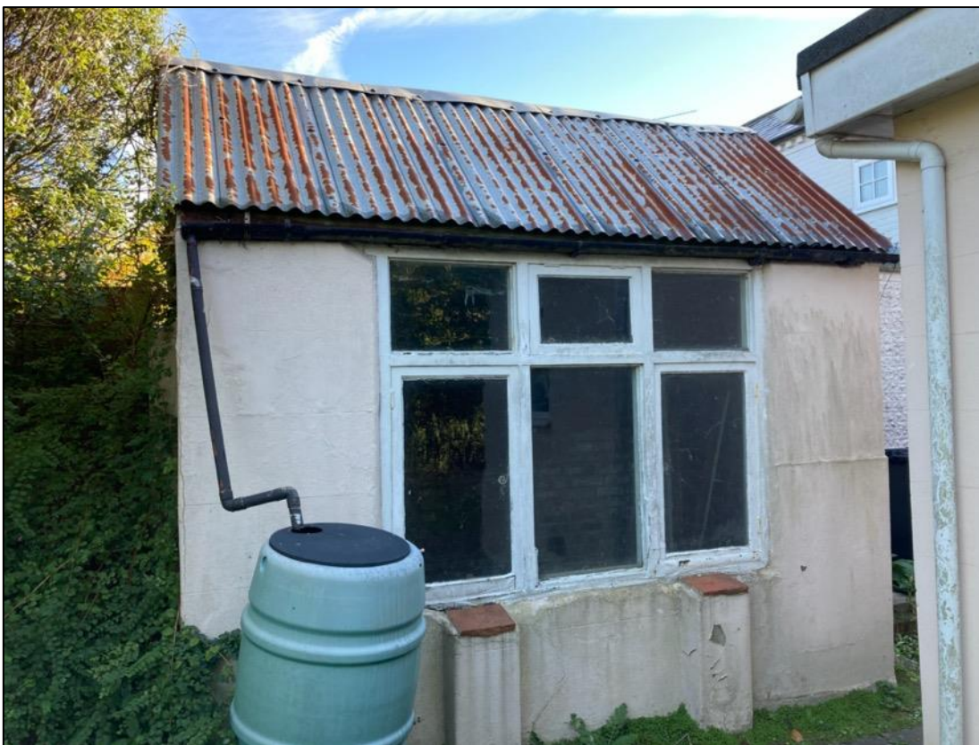
Photograph 4. Store room - exterior
