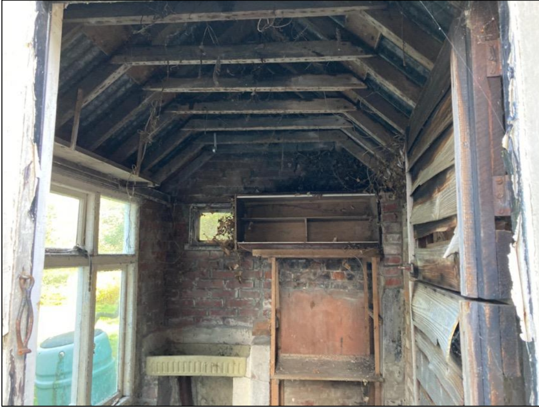
Photograph 5. Store room - interior
