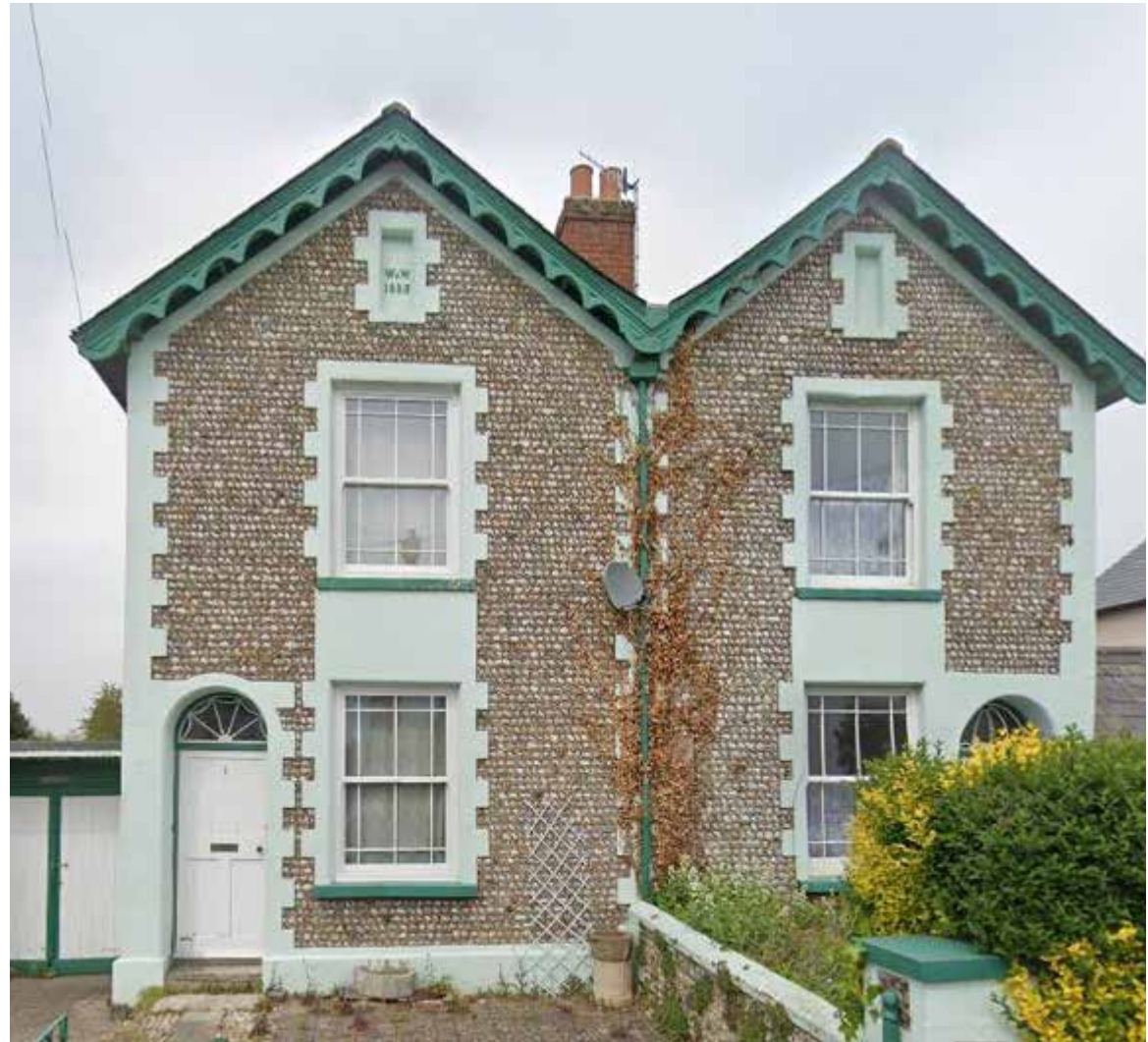
ABOVE: Nos, 1 & 2 York Road [Locally Listed]
