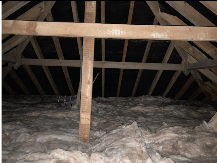
Photograph 1: Northern section of the roof void.
