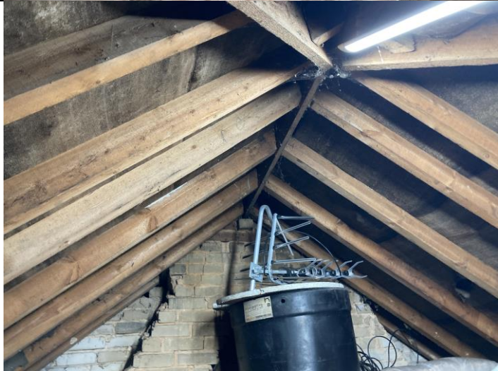
Photograph 2: Southern section of the roof void.
