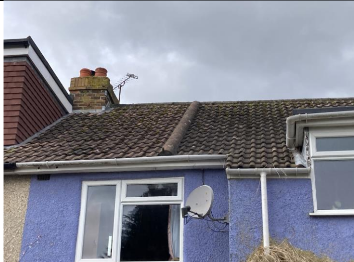
Photograph 4: Eastern facing aspect of the roof.
