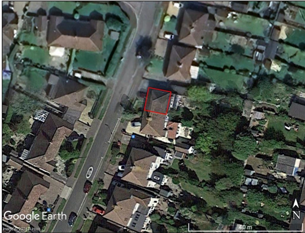
Figure 1: Satellite image indicating the inspected building and its immediate surroundings.
