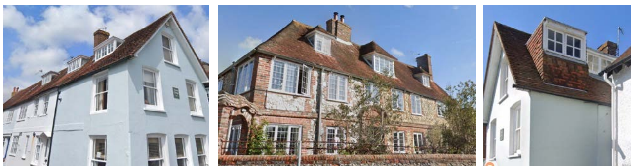
Figure 13: Examples of dormer windows and roof forms within the centre of Bosham (including on the existing terrace)
