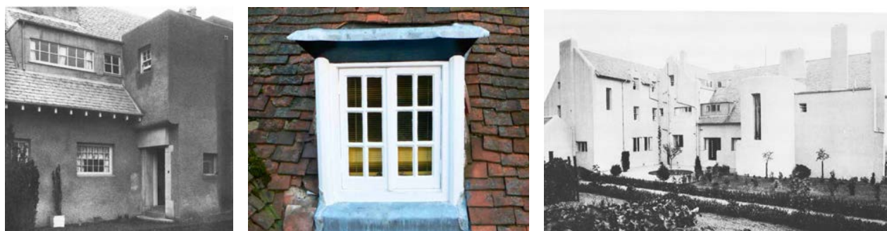
Figure 14: Examples of dormer windows on historic properties (Houses by Charles Rennie Mackintosh - Windy Hill, Kilmacolm and Hill House Helensburg)
