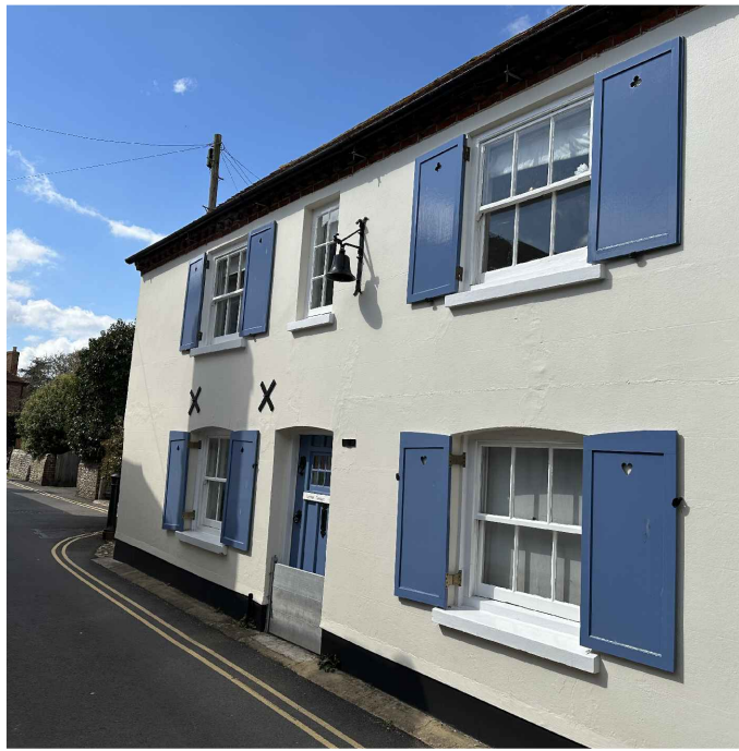
EXISTING SITE PHOTOGRAPH
