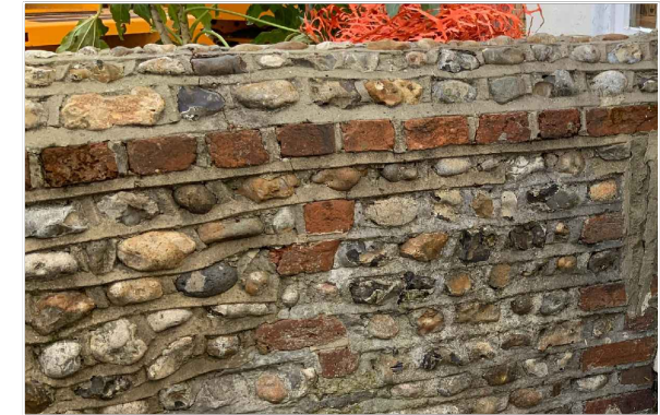
Photo: Flint / Brick Wall to be retained
