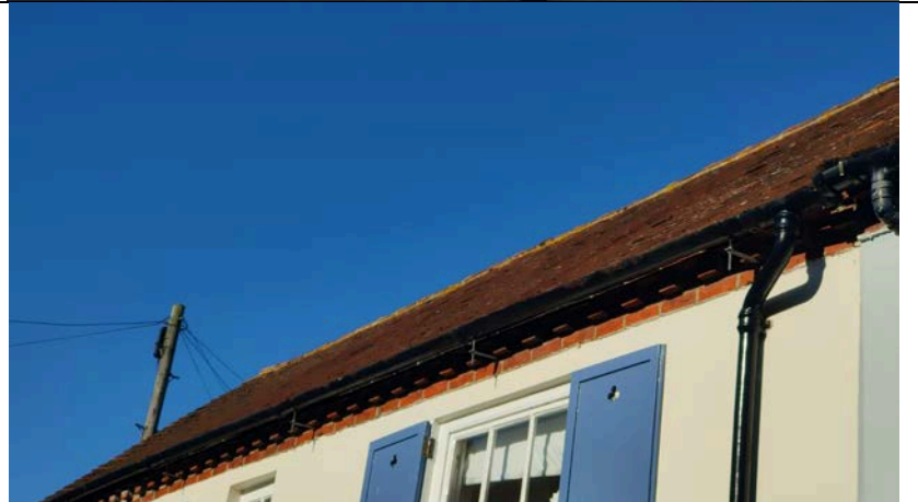
Photograph 6: Southern aspect of the roof from street level
