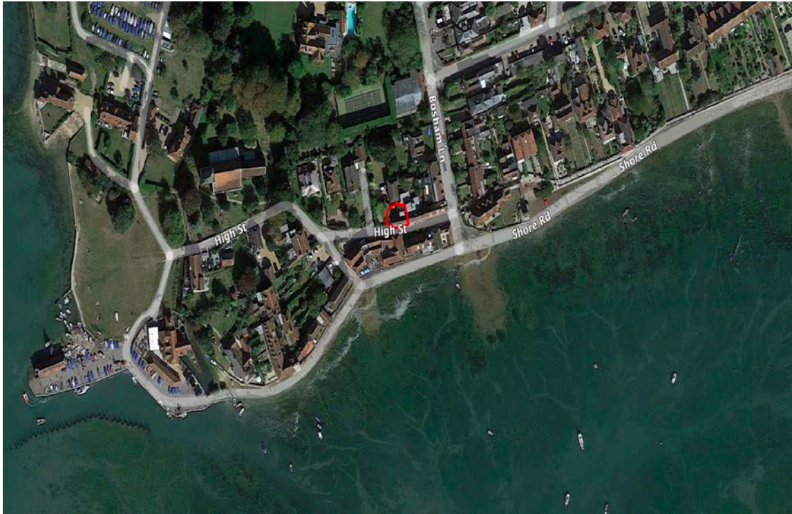
Figure 1: Satellite image indicating the surveyed building in the wider landscape. Taken from Google Earth Pro 07/02/2023
