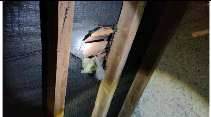
Photograph 2: Photo highlighting a potential access point in the felt to the void.
