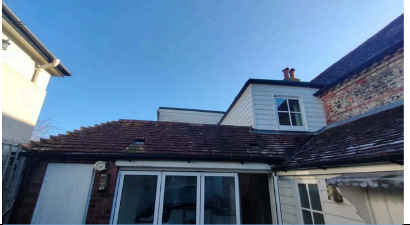
Photograph 4: Overview of the western aspect showing the existing extension
