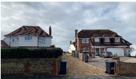
Existing driveway view from Clayton Road
