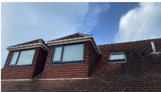
Existing red roof tiles
