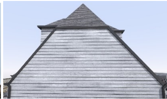
After Chimney removal
