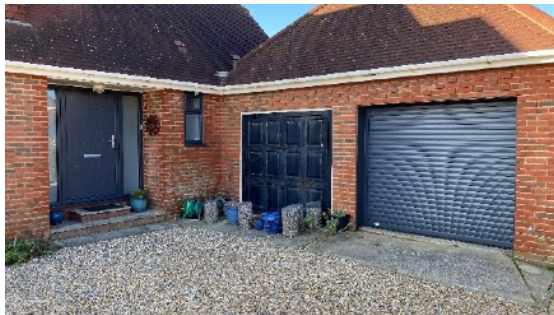
Existing front entrance
