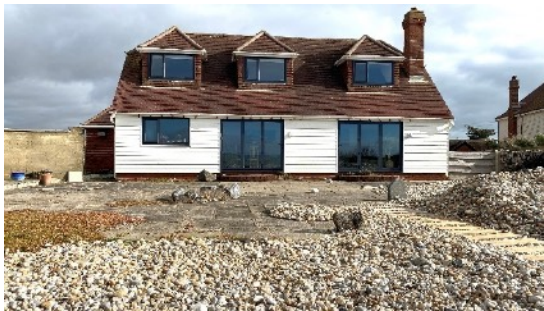
Existing rear of property
