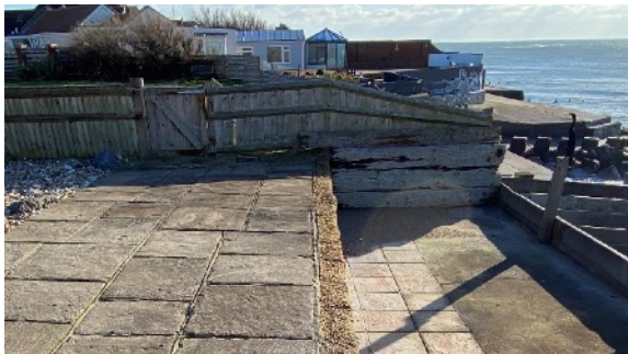
Existing sunken seating area
