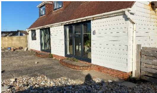
Existing rear of property
