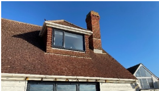
Existing dormer window
