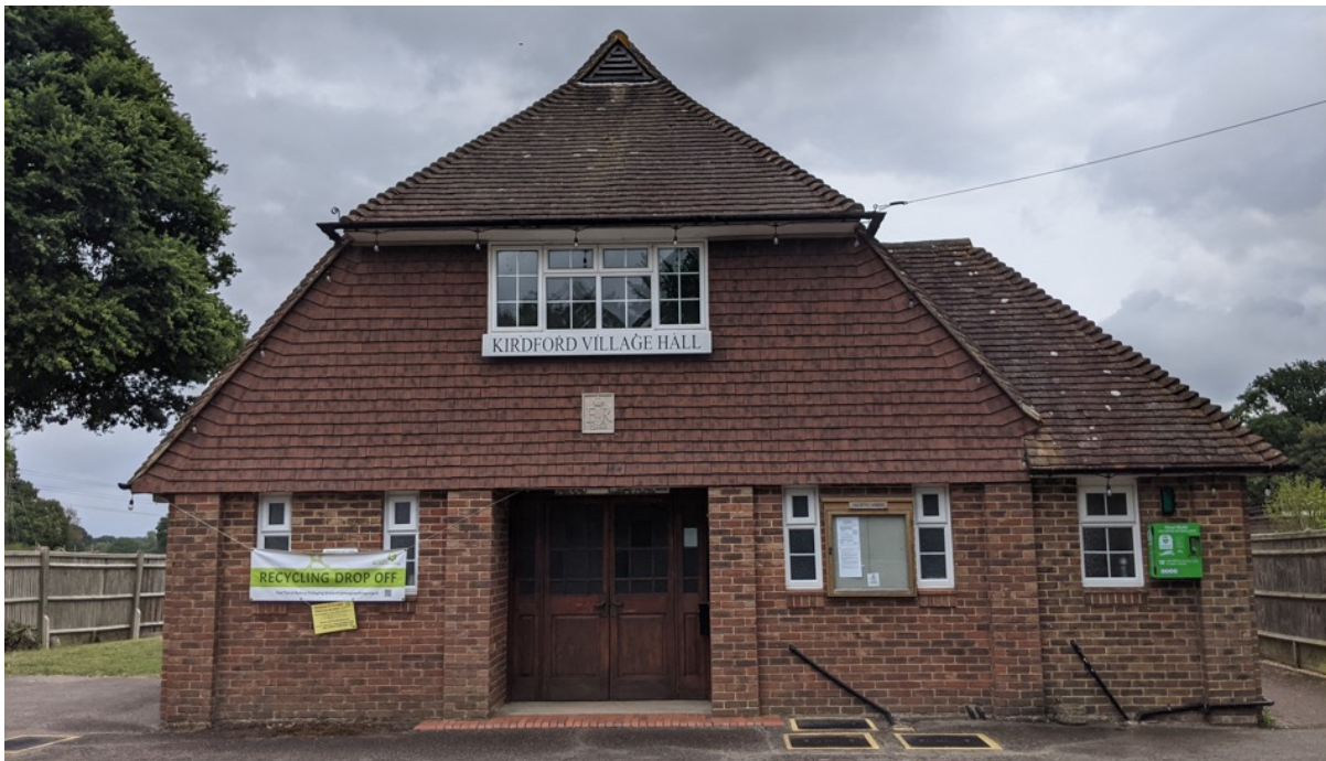
Photograph 1. The western elevation of Kirdford Village Hall.
