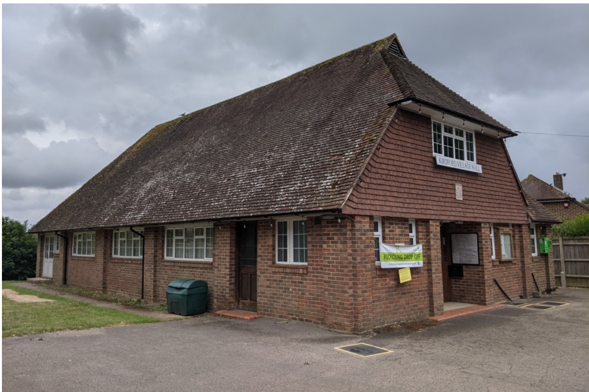
Photograph 3. The northern and western elevations.
