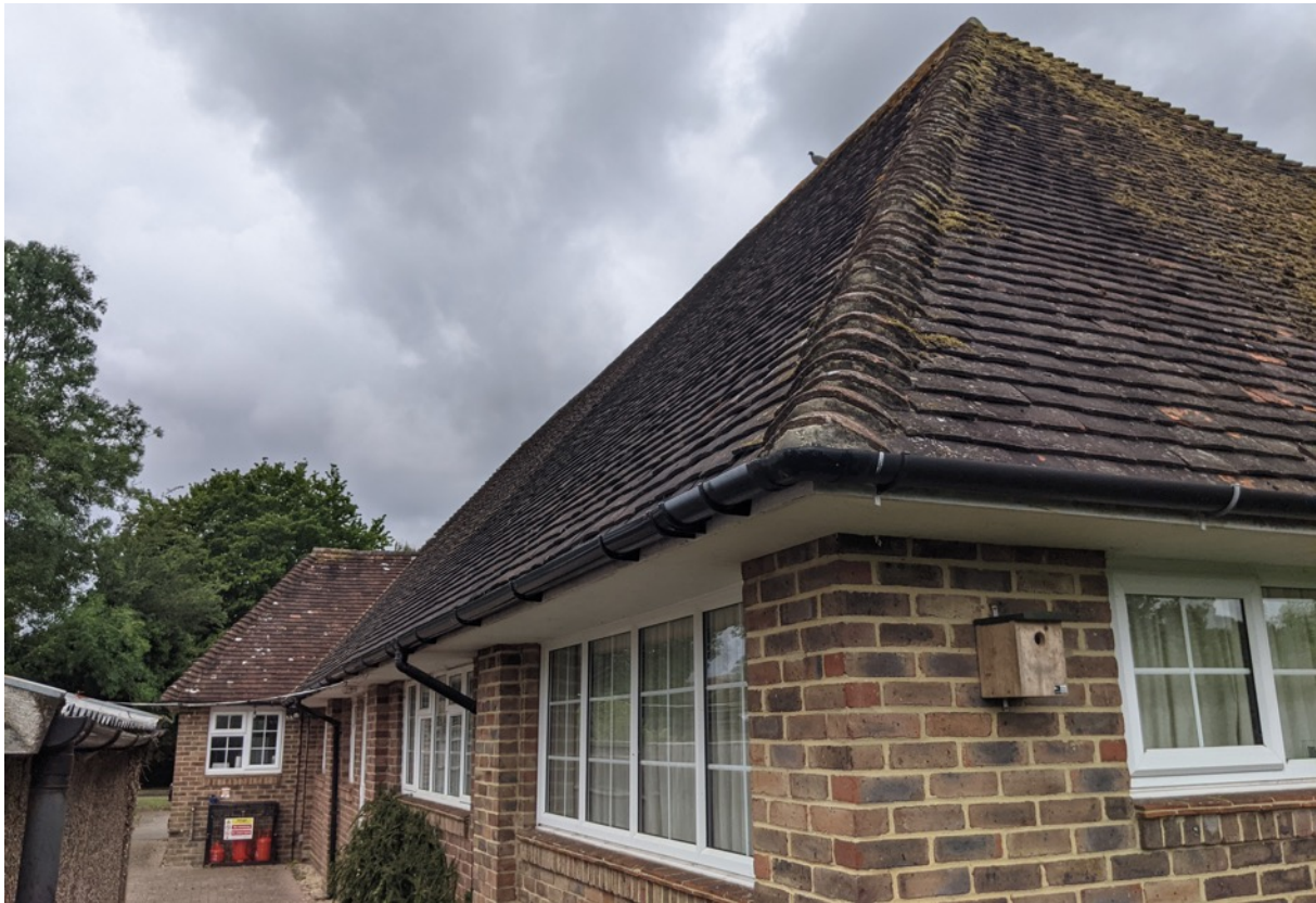
Photograph 2. The southern elevation and eastern elevations of Kirdford Village Hall.
