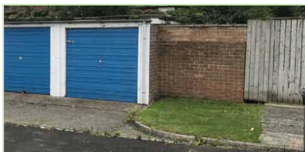
Plate 1 –Small Area of Soft Landscaping
