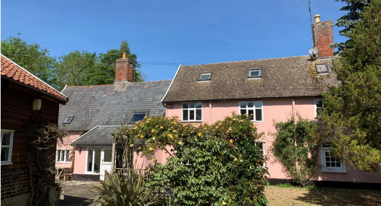
View of South East (rear) elevation of farm house.
