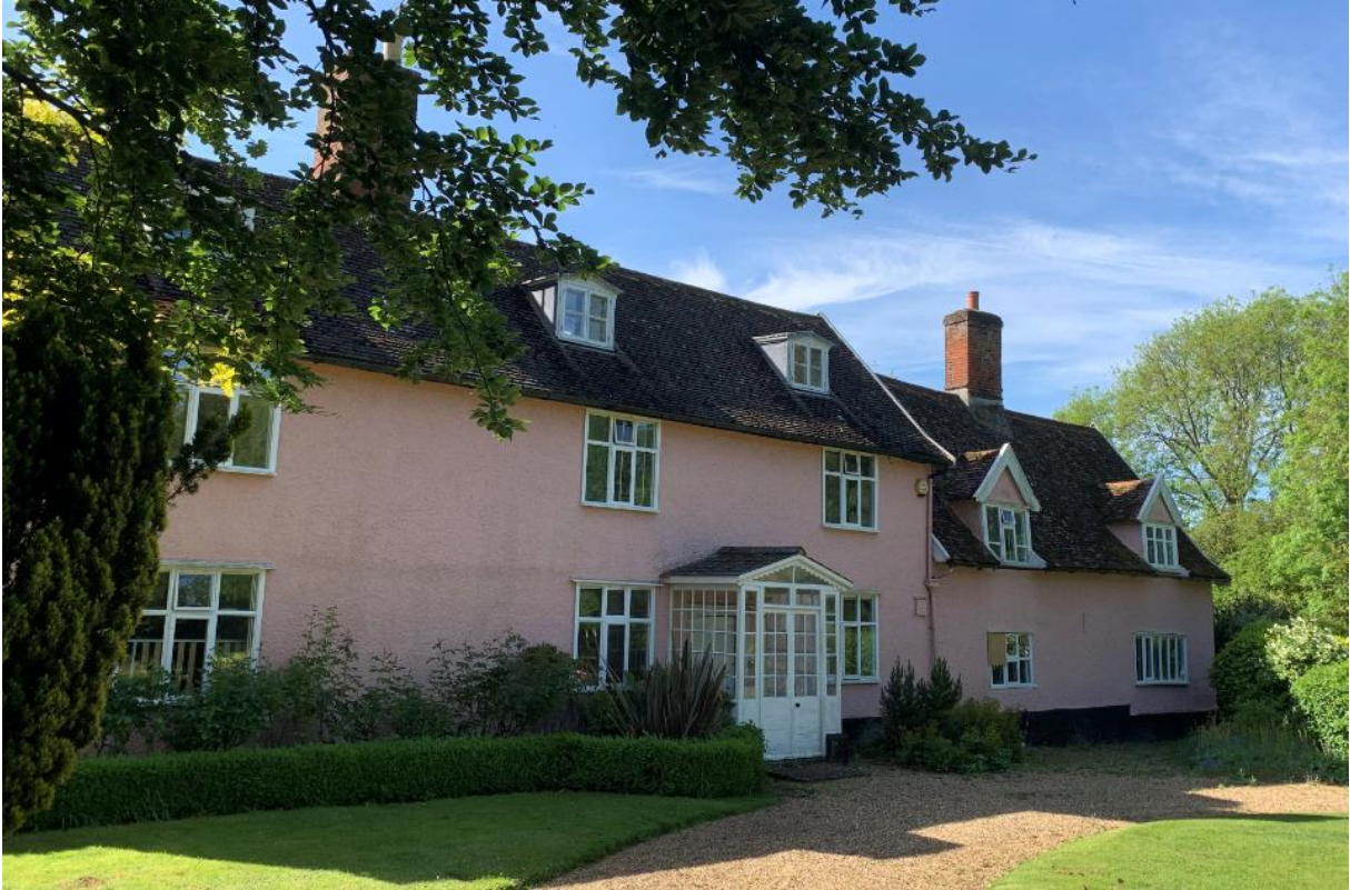
View of South East (rear) elevation of farm house.
