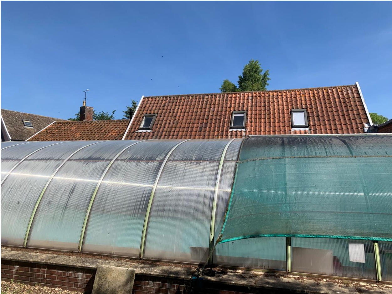
View of South West (front) elevation of farm house.
