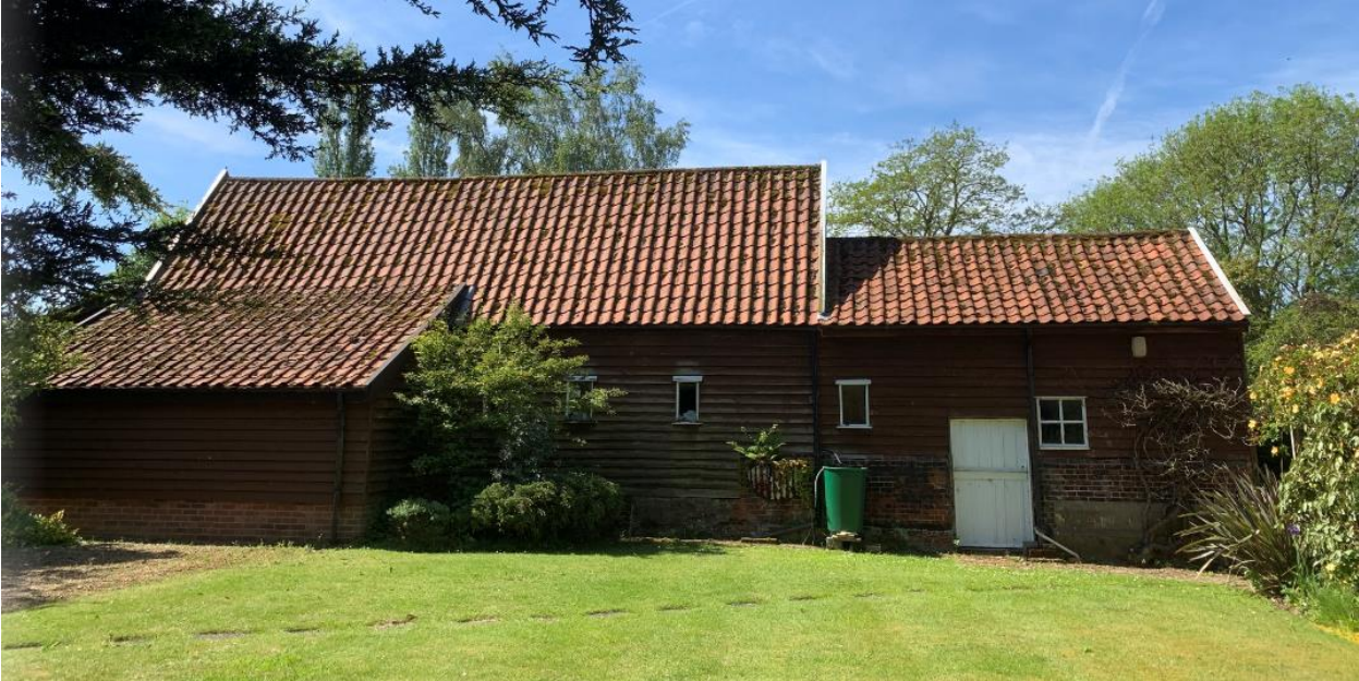
View of North East (front) elevation of barn (left) and stable (right).
