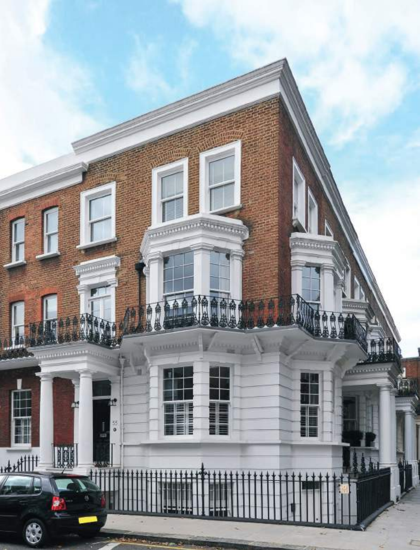
Complete new sash windows manufactured and installed.
