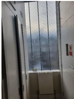
C. Rear lift shaft
