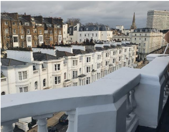
View to Gloucester Terrace from front balcony
