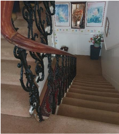
Staircase from 1st to 2nd floor
