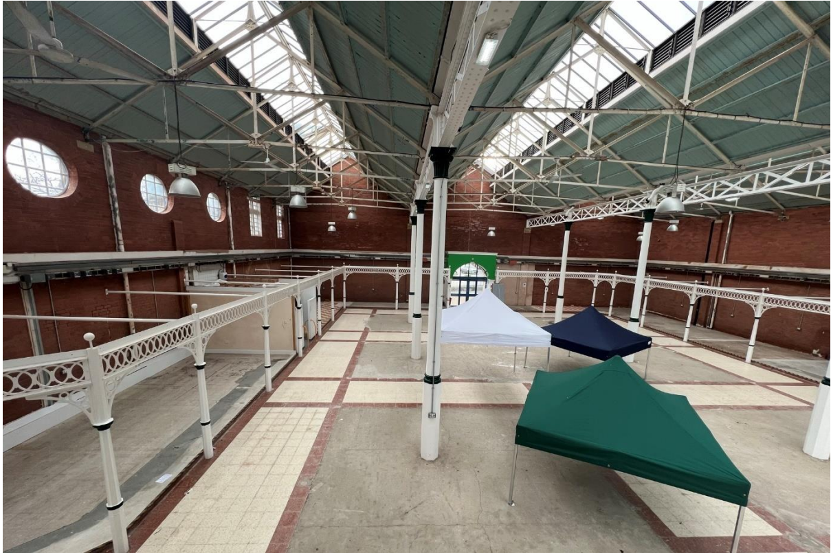
Plate 4: Interior looking south from the mezzanine
