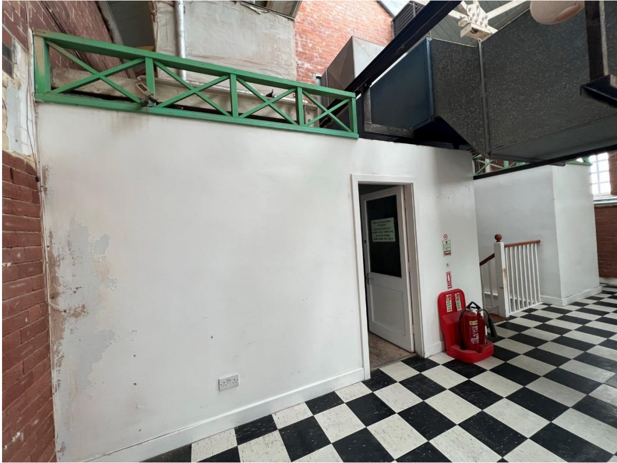
Plate 6: Office pods built into the mezzanine with stairs down
