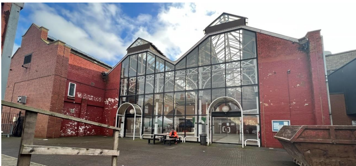
Plate 3: Modern glazing has been inserted across much of the north face
