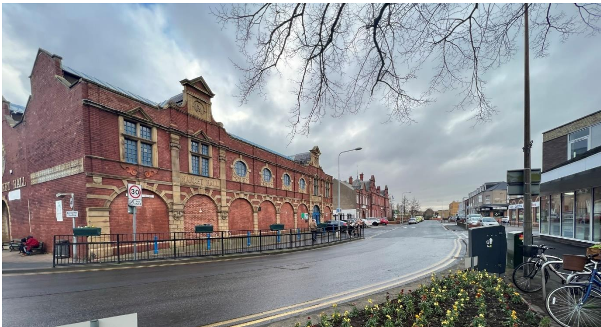
Plate 7: View along Estcourt Terrace showing relationship with the Grade II listed Police Station and former Magistrates' Court in the distance
