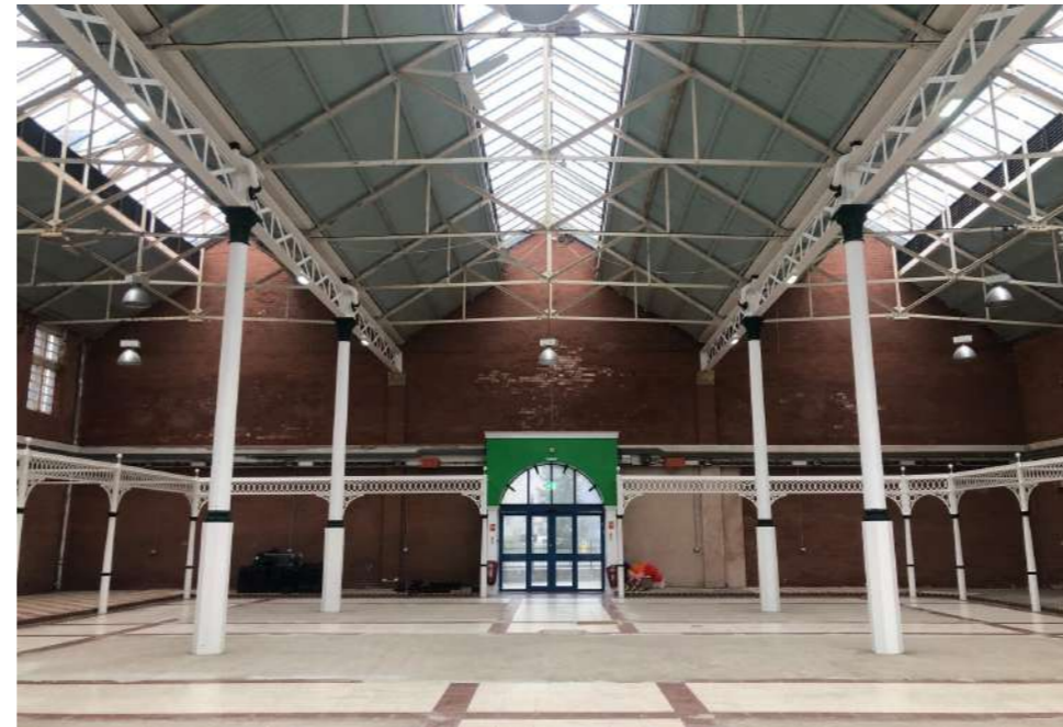
VIEW LOOKING SOUTH TOWARDS MAIN ENTRANCE
