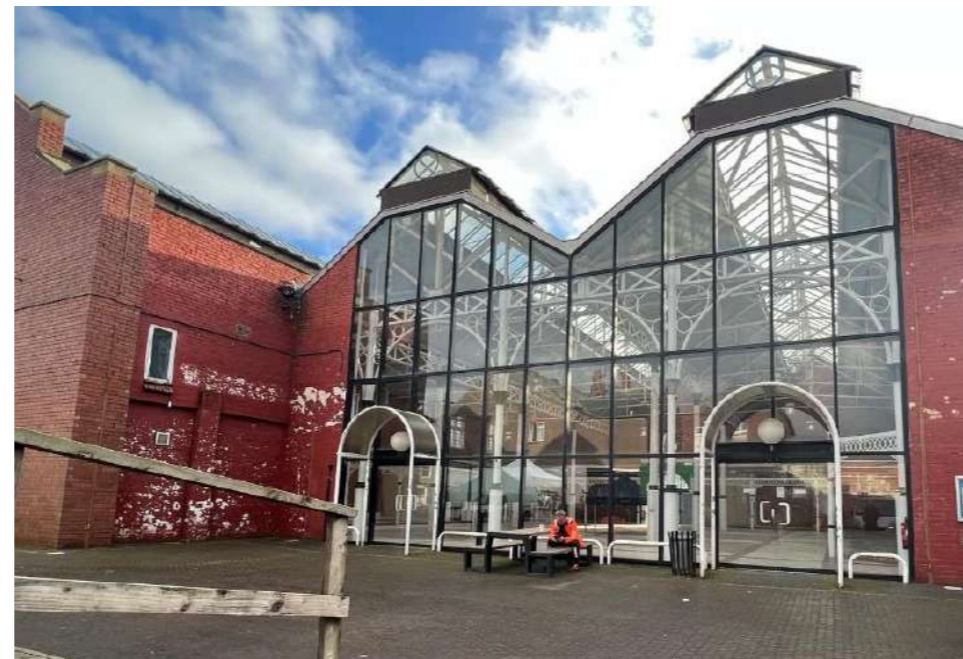
GLAZING TO NORTH ELEVATION / VIEW FROM YARD
