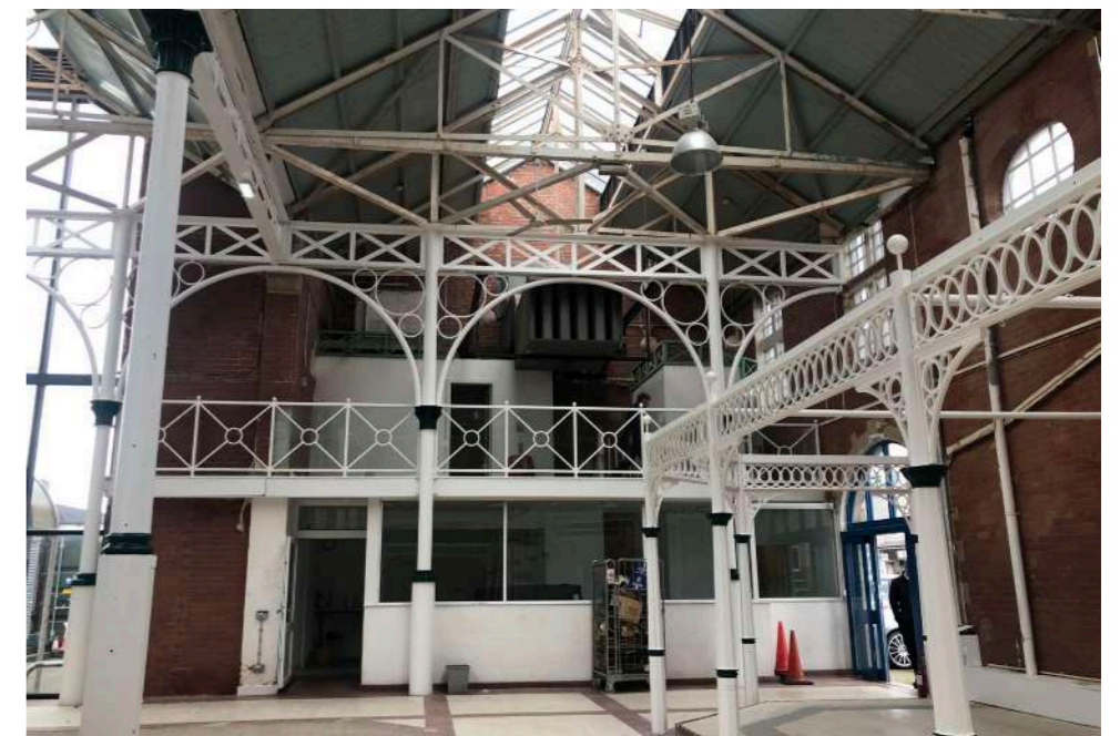
VIEW OF ANCILLARY SPACES IN THE BAY
