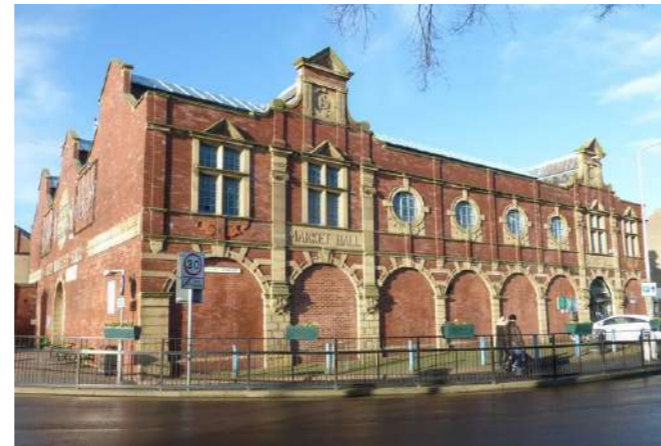
EXISTING PHOTOGRAPH OF EAST ELEVATION
