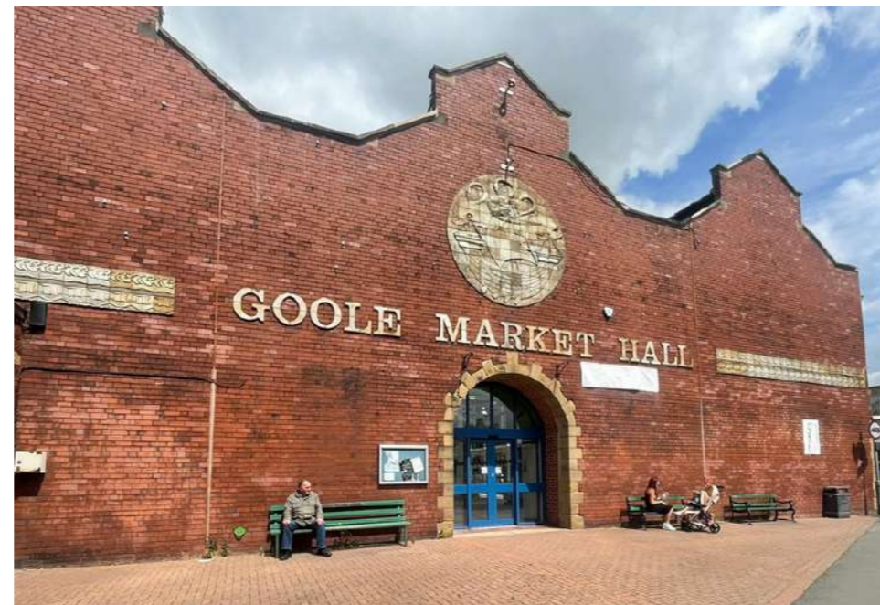
'FRONT' SOUTH ELEVATION / APPROACH FROM BOOTHFERRY ROAD
