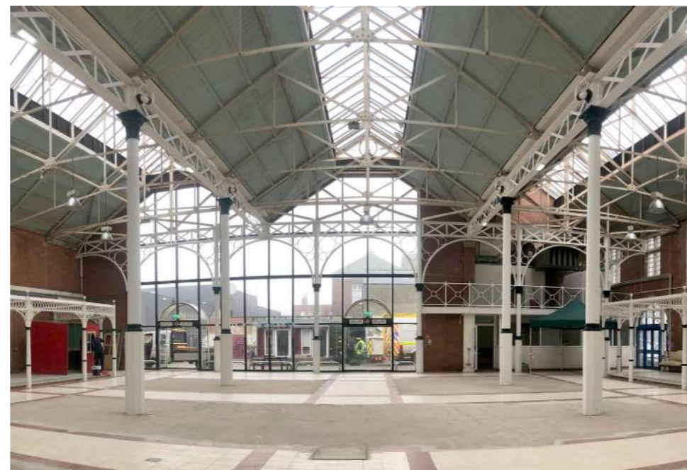
VIEW LOOKING NORTH TOWARDS GLAZING & YARD
