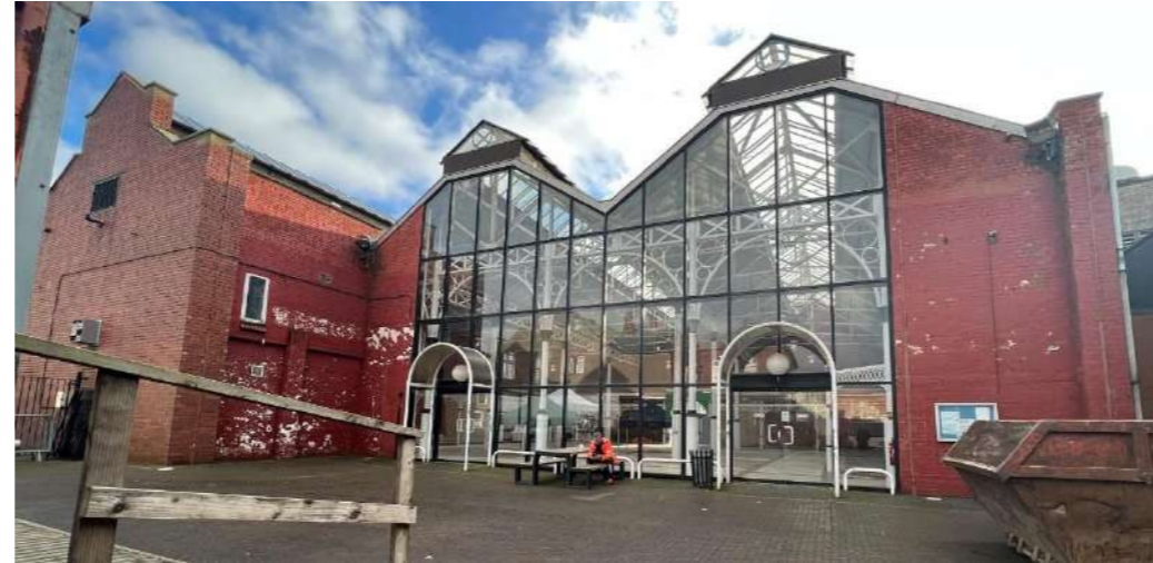
PHOTOGRAPH OF EXISTING NORTH ELEVATION
