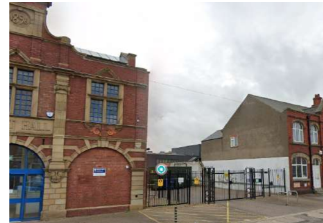
EXISTING PHOTOGRAPH OF SECURITY GATE
