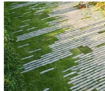
DYNAMIC PERMEABLE PAVING
