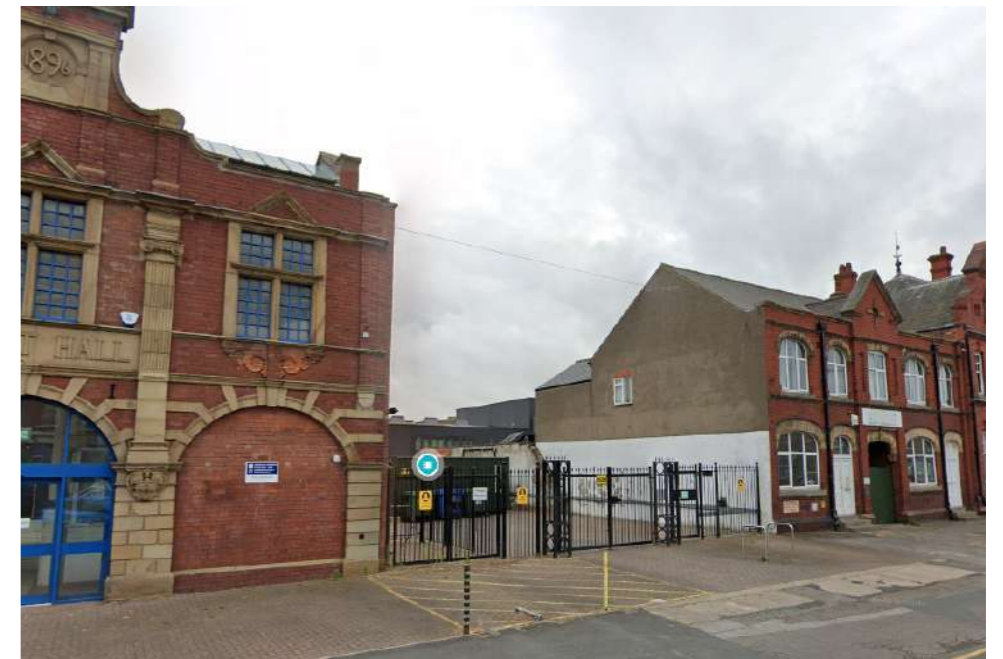
VIEW OF SECURITY GATE & YARD FROM ESTCOURT TERRACE ROAD
