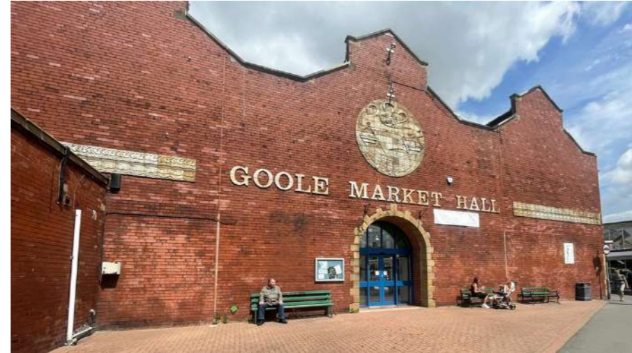
PHOTOGRAPH OF EXISTING SOUTH ELEVATION
