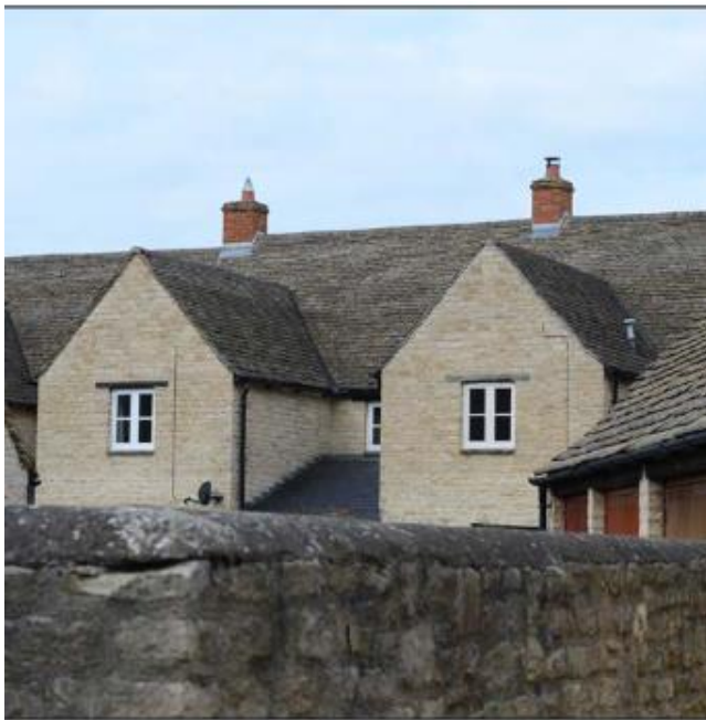
Figure 1 - Rear 2 storey extensions
