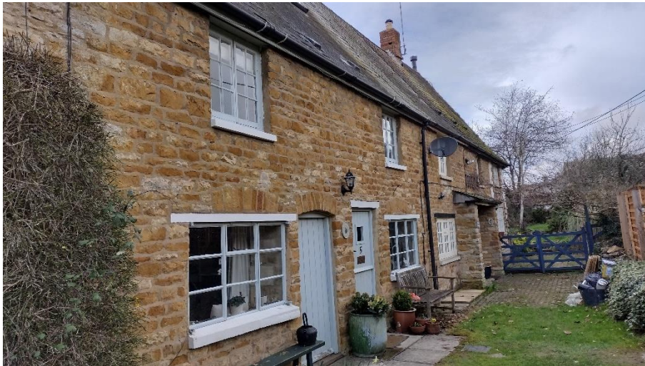
Main elevation of house
