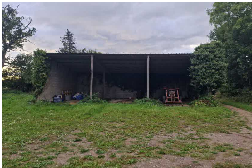
Photo 1: The front of the open barn, the south-east aspect
