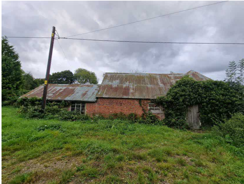
Photo 7: The old stables showing the brick-built construction, southern aspect
