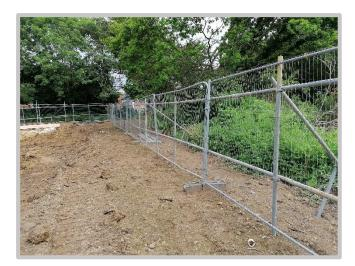
The default specification should consist of a vertical and horizontal scaffold framework, well braced to resist impacts. The vertical tubes should be spaced at a maximum interval of 3 m and driven securely into the ground. Onto this framework, welded mesh panels should be securely fixed.
