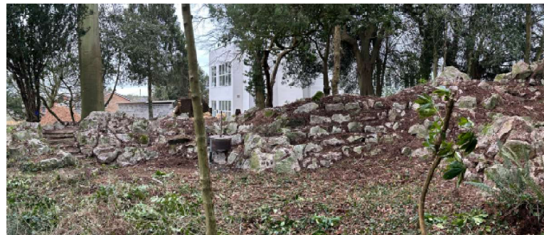
Former Rockery Existing Condition
