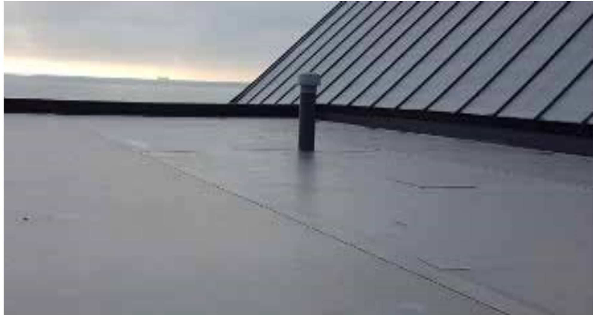
Fig 13.1 Single PVC Membrane Roofing System
