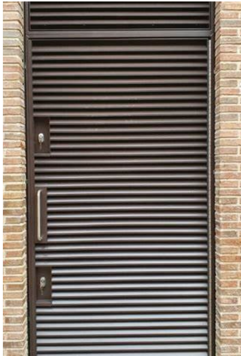
Fig 6.1: External Metal Louvre Doors
