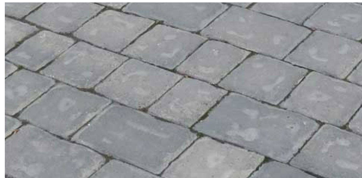
Fig 17.2: Medium Grey Concrete Setts Paving
