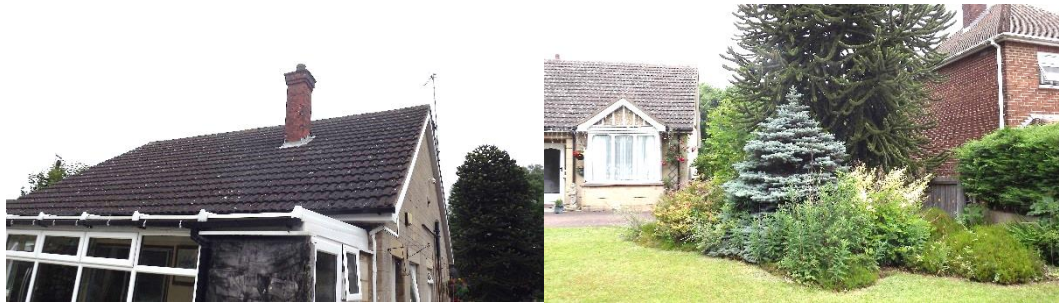
Northern elevation of B1 and conservatory (left) (right) southern boundary garden
