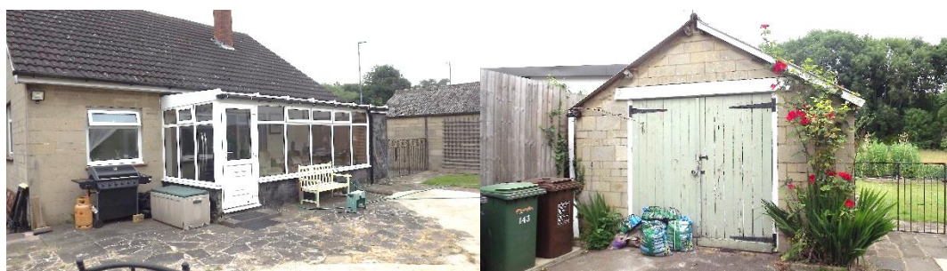
Figure 4.0 (left) B1 northern elevation and uPVC extension Figure 5.0 (right) detached garage B2
