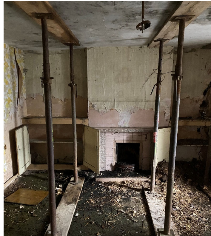
Cottage 2 props to ceiling in living room
