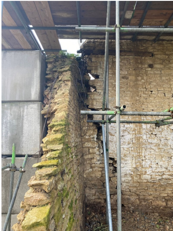
Cottage 2/barn part wall/gable end with rear wall separated
