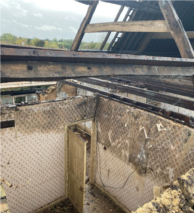
Cottage 2 removed section of roof
