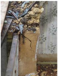
The wall head should be cleared on both the north-west and south-eastern side from the scaffold, ensuring adequate protection/handrail on the inside face. The propped first floor can then be accessed and the fallen masonry cleared. The birdcage should then be continued up to prop the purlins and the truss of Cottage 2, it can also be used so both sides of the gable wall are propped.
