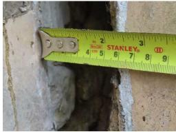
On the opposite side the ivy roots have caused noticeable damage and this will require removing and then repaired.
