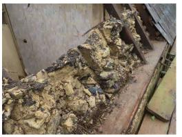
The staircase leading up to the first floor is quite poor as the bottom treads have collapsed and these should either be removed or made good so that safe access can be provided.
