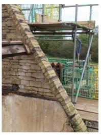
At the junction with Cottage 1, the purlins span between trusses which are located in the middle of each property. The purlins should be propped off the central party wall so that the roofs of Cottage 1 and Cottage 2 are independently supported.
