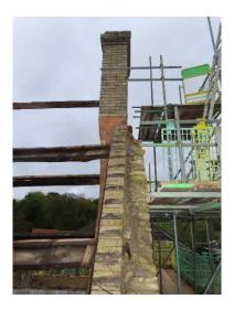
The first floor is currently propped but there is stonework from the south eastern window which has collapsed onto the floor where the lintol has failed. The reveal and wall head are also loose and likely to fall. The first floor should be fully propped by either supplementing the existing props or utilising the proposed bird cage which is required to be built.
