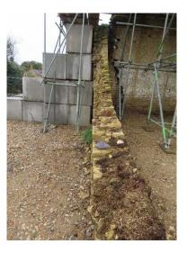
It is evident that the concrete buttress blocks are working as the wall is now leaning hard against them.
