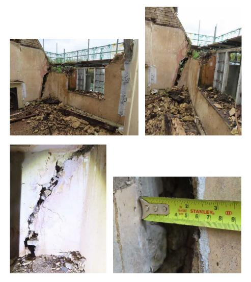
On the opposite side the ivy roots have caused noticeable damage and this will require removing and then repaired.
