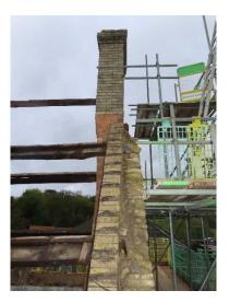
The first floor is currently propped but there is stonework from the south eastern window which has collapsed onto the floor where the lintol has failed. The reveal and wall head are also loose and likely to fall. The first floor should be fully propped by either supplementing the existing props or utilising the proposed bird cage which is required to be built.
