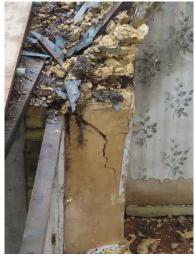
The wall head should be cleared on both the north-west and south-eastern side from the scaffold, ensuring adequate protection/handrail on the inside face. The propped first floor can then be accessed and the fallen masonry cleared. The birdcage should then be continued up to prop the purlins and the truss of Cottage 2, it can also be used so both sides of the gable wall are propped.
