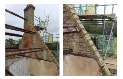
At the junction with Cottage 1, the purlins span between trusses which are located in the middle of each property. The purlins should be propped off the central party wall so that the roofs of Cottage 1 and Cottage 2 are independently supported.
