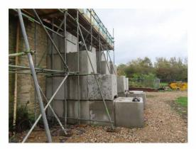
The rafters from Cottage 2 have been removed as the wall-plate had displaced excessively as noted previously. The purlins are still built into the gable which is advantageous to aid restraint.
