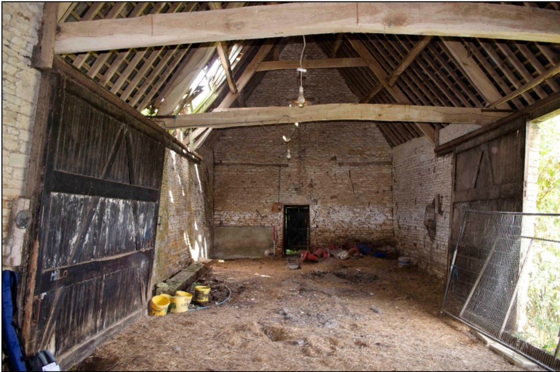
Appendix 2.43 View of room IG9 Barn I, looking north-east (2018)
