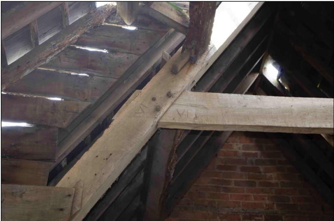
Appendix 2.58 Detail of truss above room 2G1, Barn 2, looking north-west (2018)
