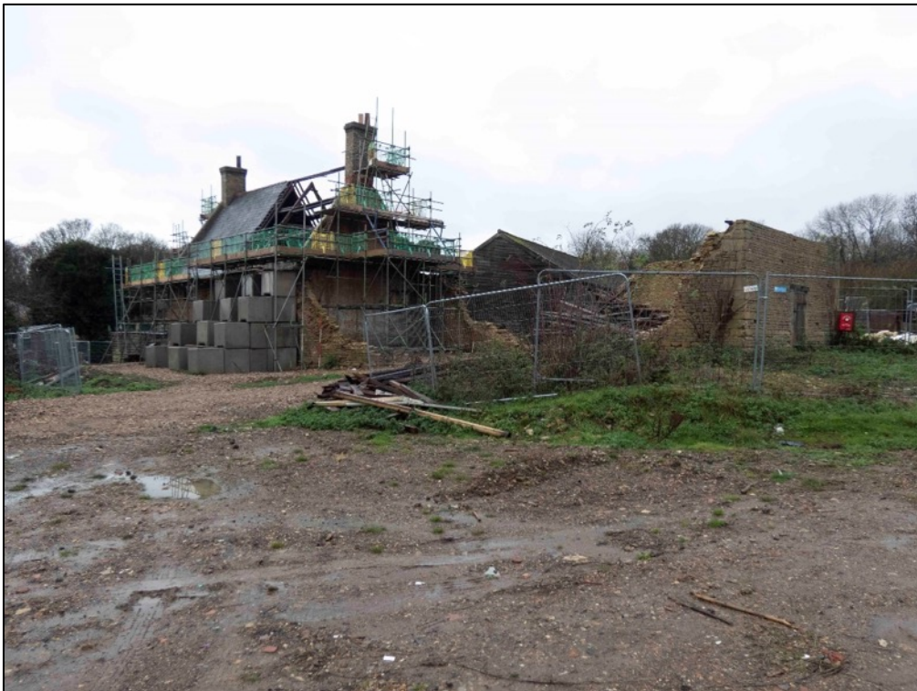
Appendix 2.10 View of Cottages 1 & 2 and Barn 1, looking west (2023)
