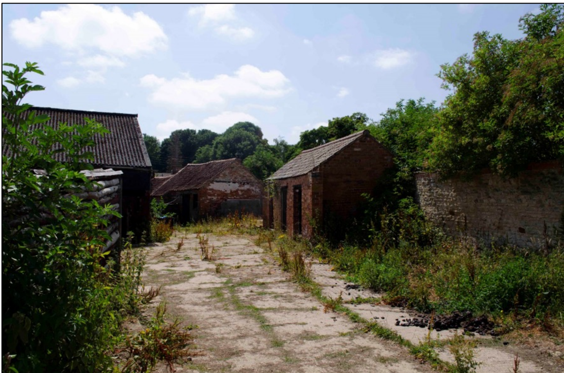
Appendix 2.4 View looking south-east into the farm yard, showing the outbuildings (2018)
