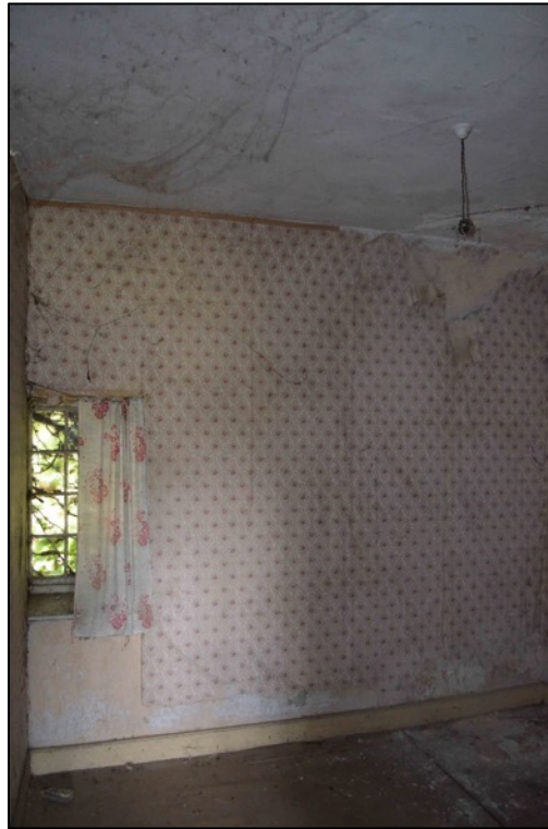
Appendix 2.21 View of room IF7 Cottage 1, looking west (2019)
