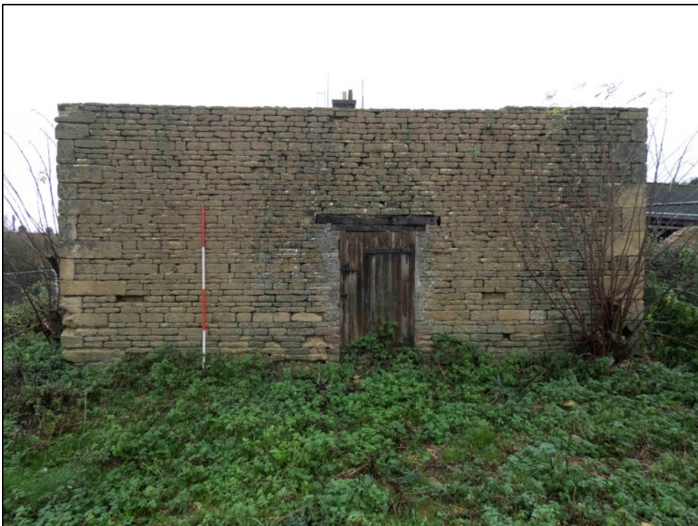
Appendix 2.38 North-east gable of Barn I , looking south-east (2023)
