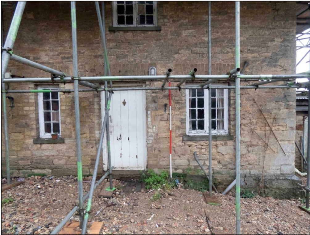
Appendix 2.7 View of north-west elevation of Cottage 2 , looking south-east (2023)
