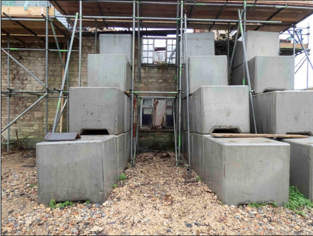
Appendix 2.13 View of south-east elevation of Cottage I , looking north-west (2023)
