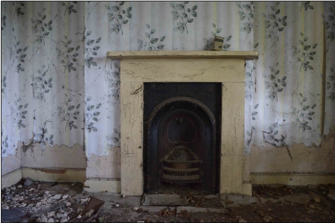
Appendix 2.19 Detail of fireplace in room IF6, Cottage I, looking north-east (2019)
