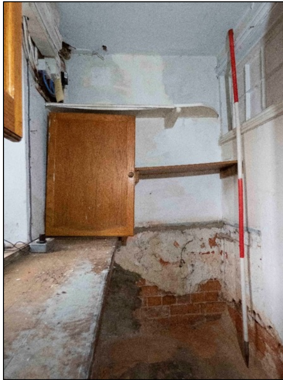
Appendix 2.25 View of room IG3 Cottage 2, looking north-east (2023)
