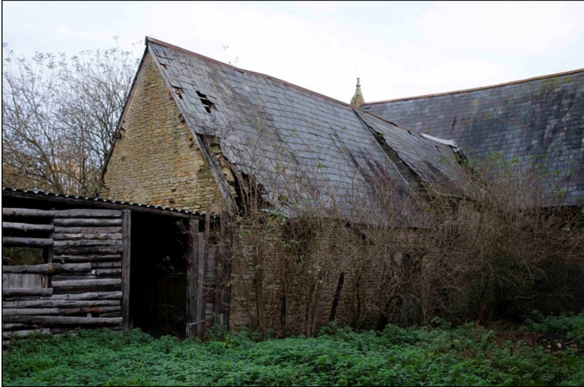
Appendix 2.47 View of Barn 2, looking east (2018)
