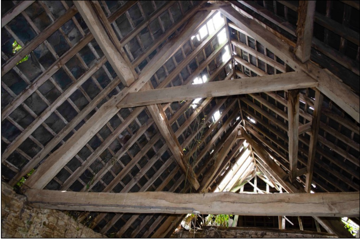
Appendix 2.57 Detail of truss above room 2G1, Barn 2, looking south-east (2018)
