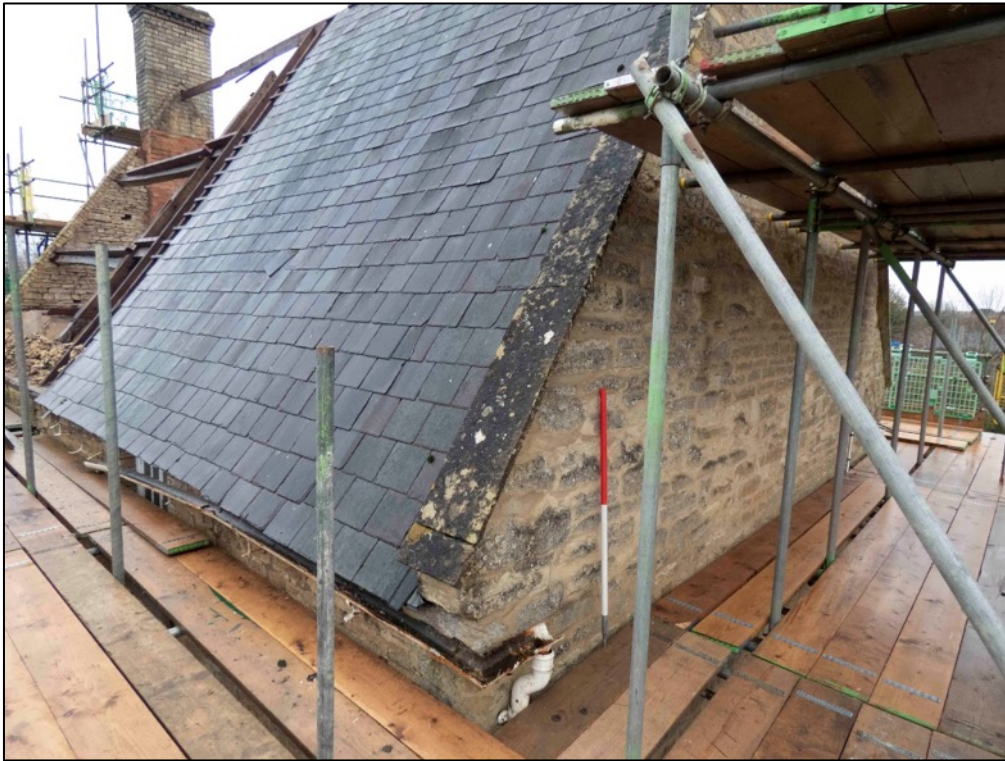
Appendix 2.31 View of roof of Cottage 2 , looking east, showing gable end (2023)
