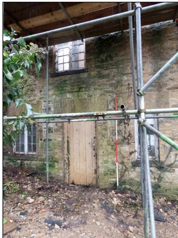
Appendix 2.6 View of north-west elevation of Cottage I , looking south-east (2023)
