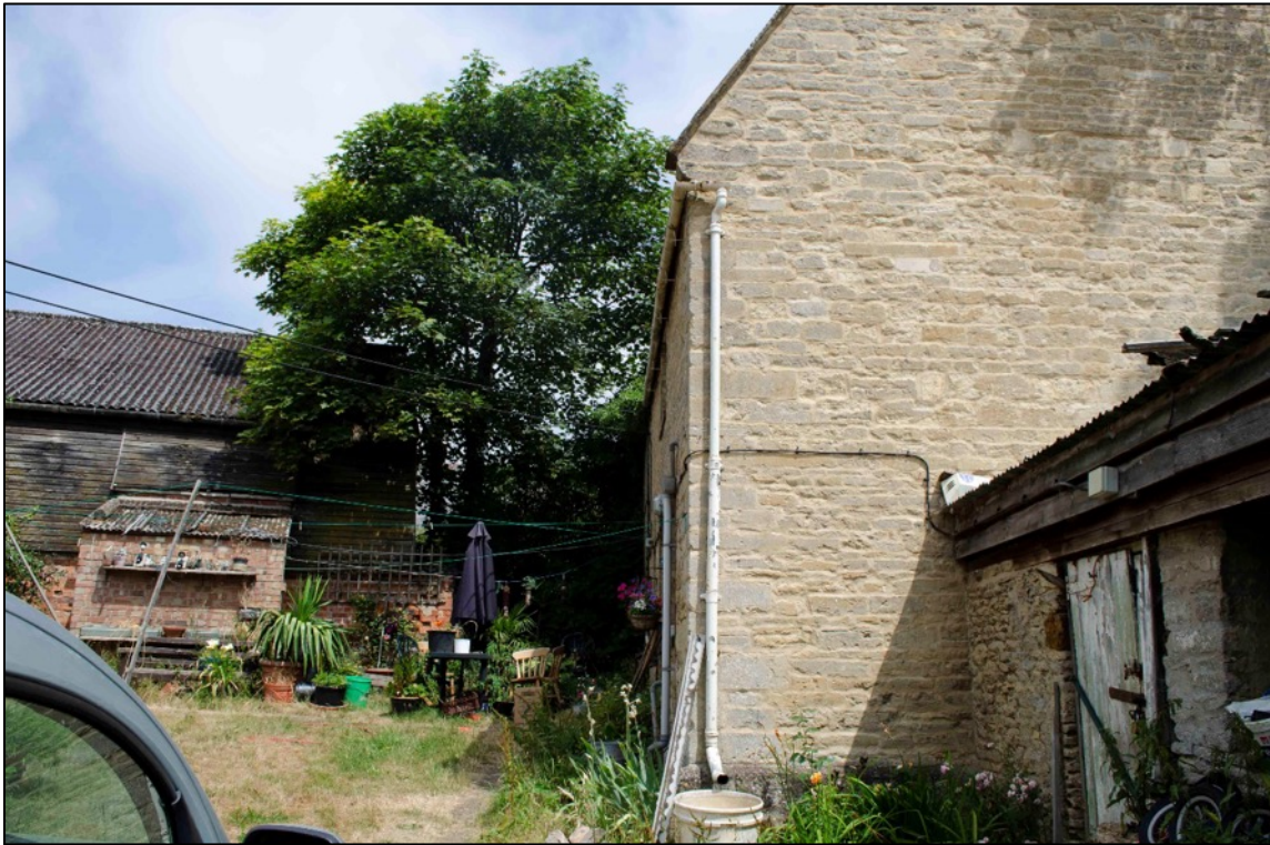
Appendix 2.3 View looking north-west along the side of Cottages 1 & 2 (2018)
