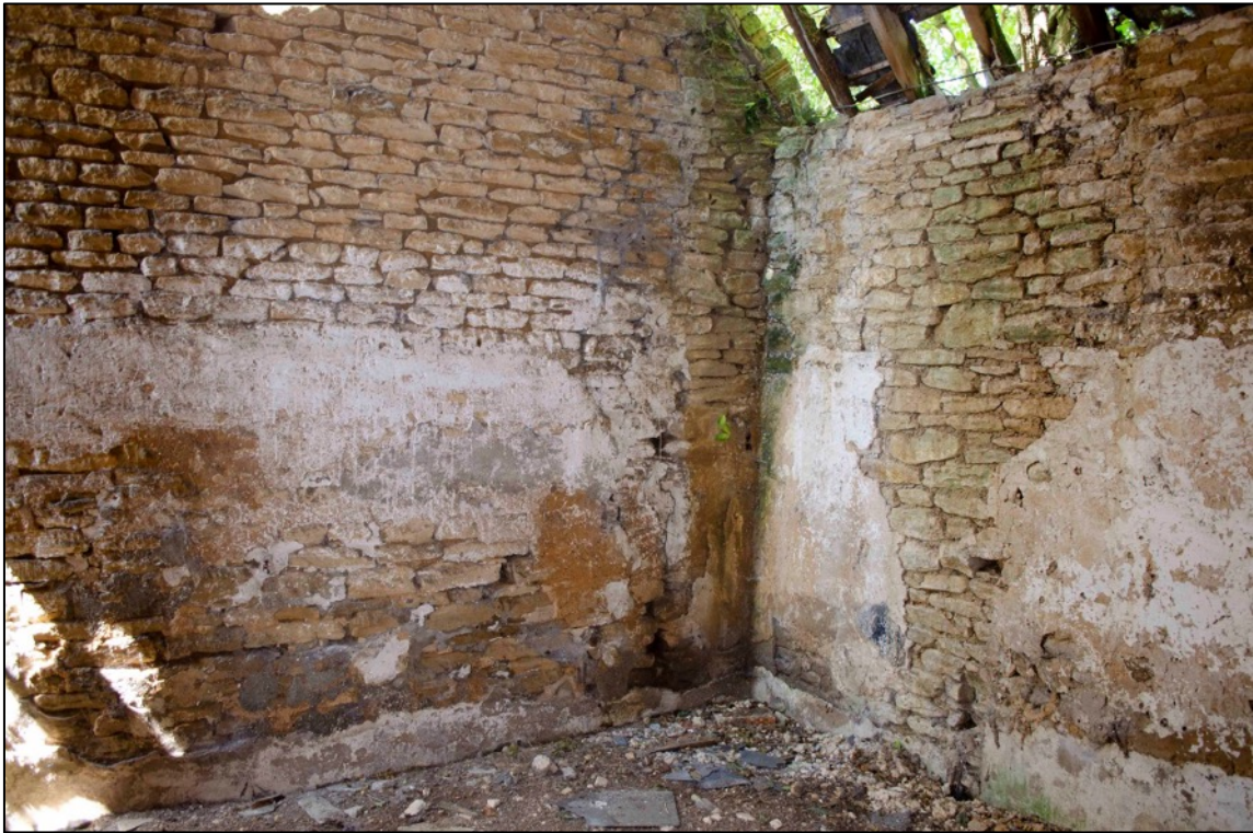
Appendix 2.53 View of room 2G2, Barn 2, looking north (2018)
