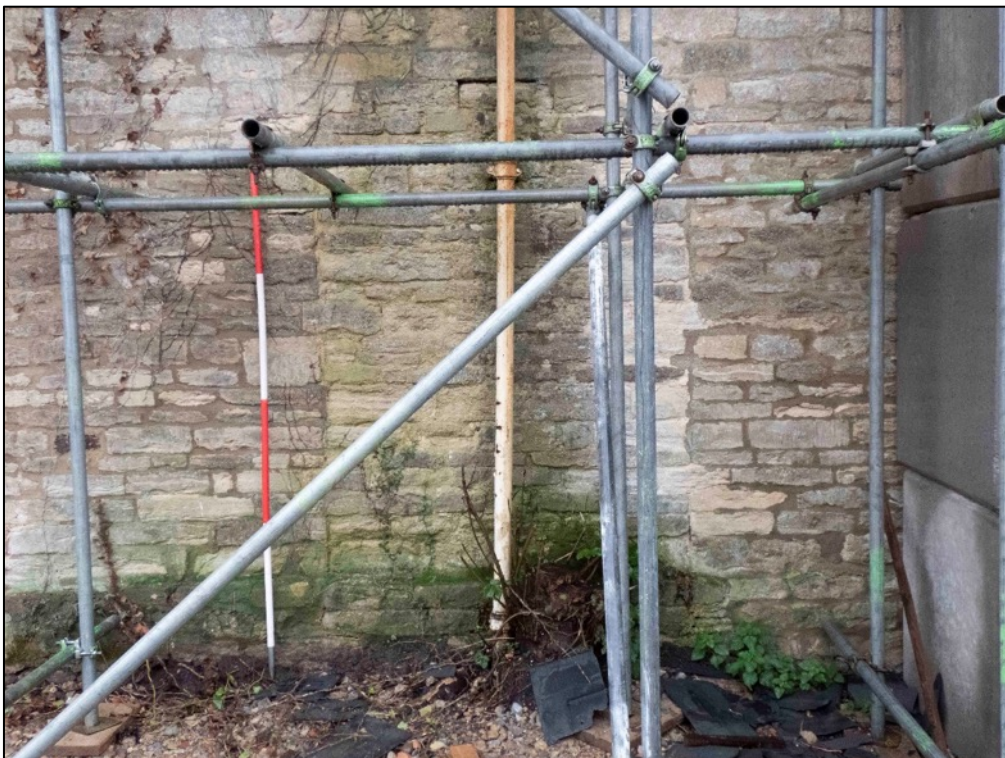
Appendix 2.12 Detail of blocked doorway in south-east elevation of Cottages 1 & 2 (2023)
