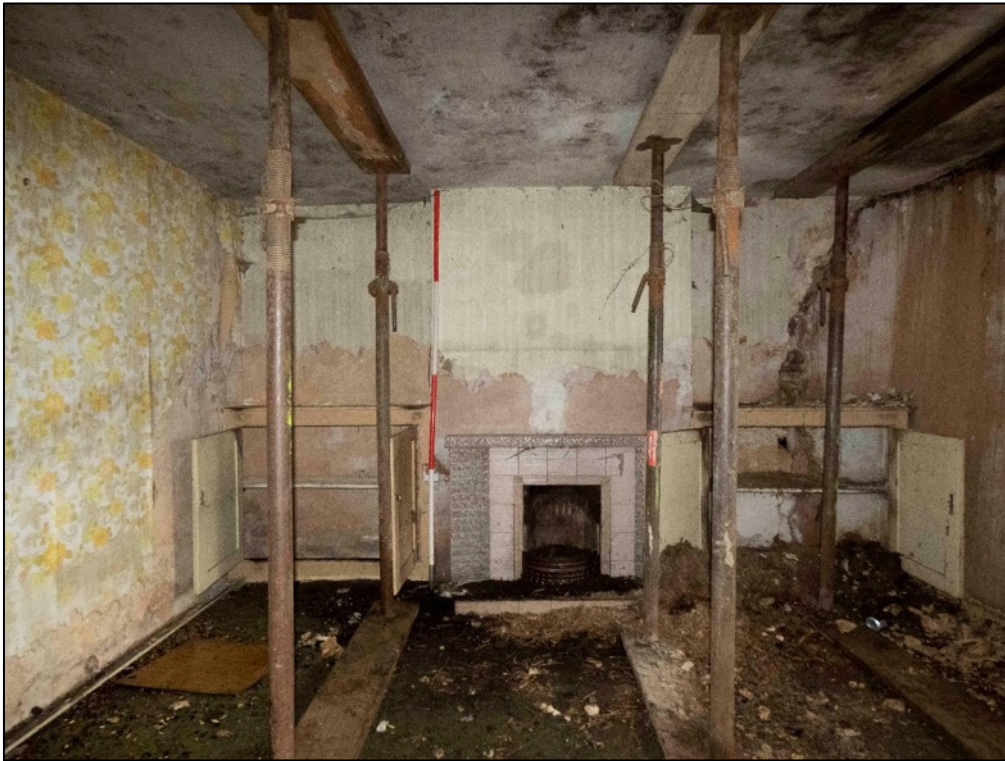
Appendix 2.15 View of room IG5, Cottage I, looking north-east (2023)
