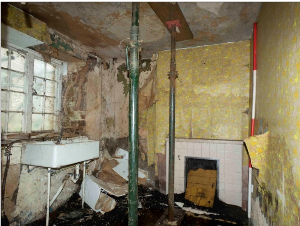
Appendix 2.14 View of room IG6 , Cottage I , looking north (2023)
