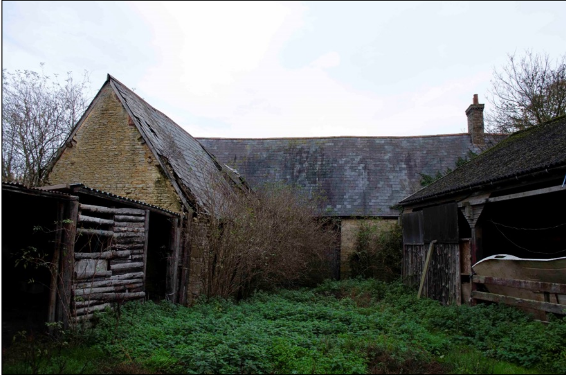
Appendix 2.5 View across the farm yard to Barns 1 and 2 , looking south-east (2018)
