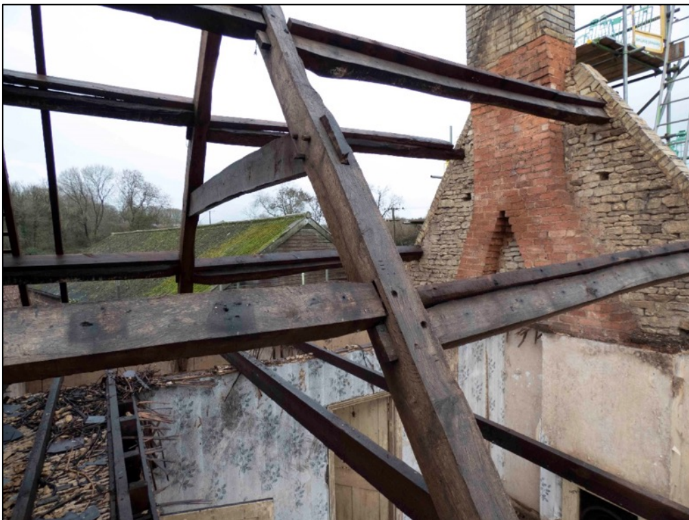
Appendix 2.34 Detail of truss above Cottage I , looking north
