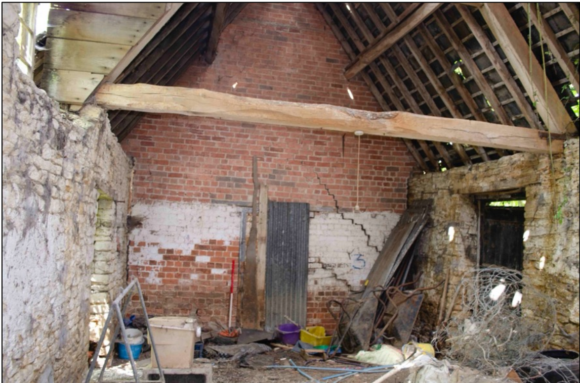
Appendix 2.52 View of room 2G1, Barn 2, looking north-west (2018)
