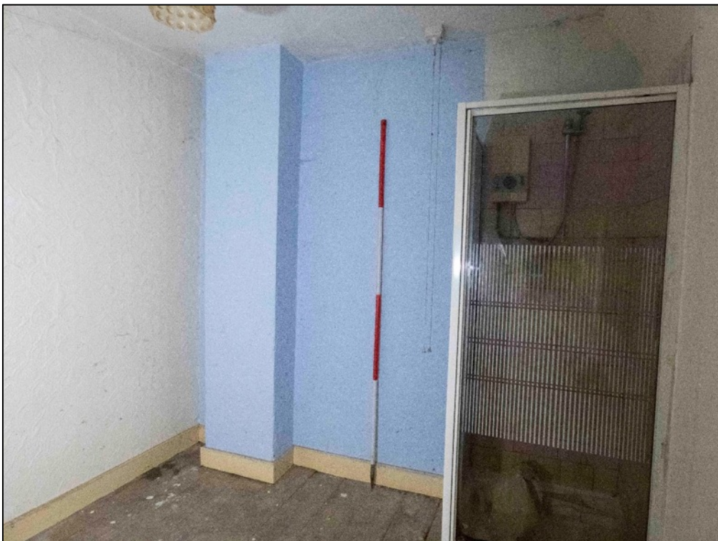
Appendix 2.30 View of room IF3 Cottage 2, looking south-west (2023)
