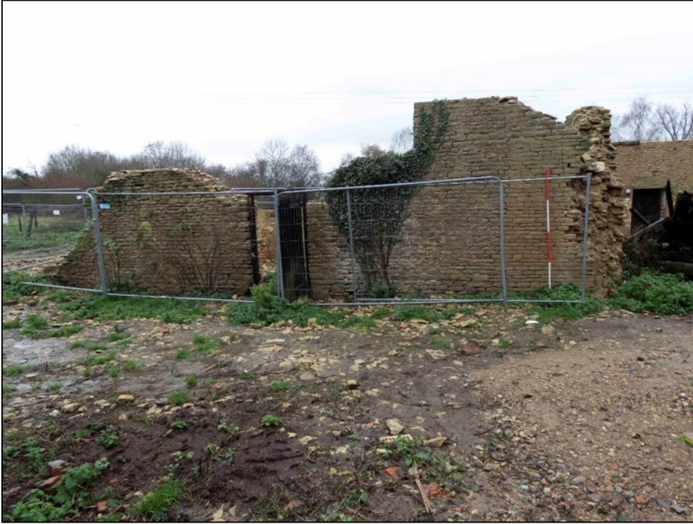
Appendix 2.49 View of Barn 2, looking north-west (2023)
