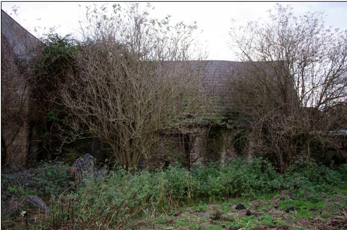
Appendix 2.50 View of Barn 2, looking south-east (2018)
