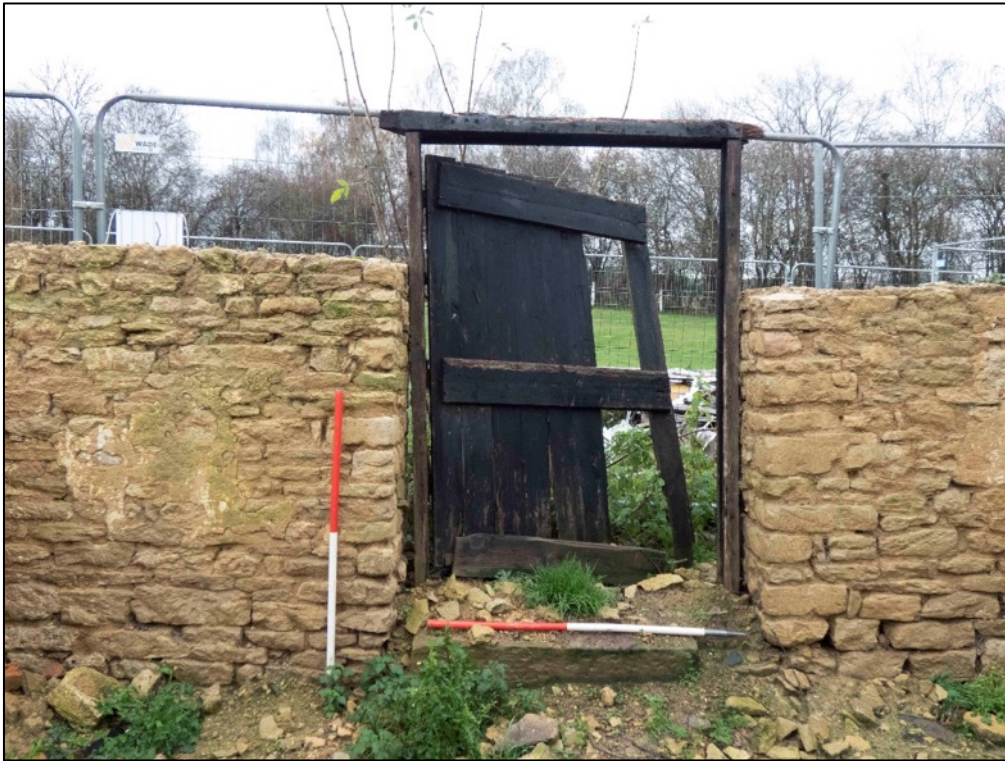
Appendix 2.55 Detail of door in north-east wall of room 2G1, Barn 2 (2023)
