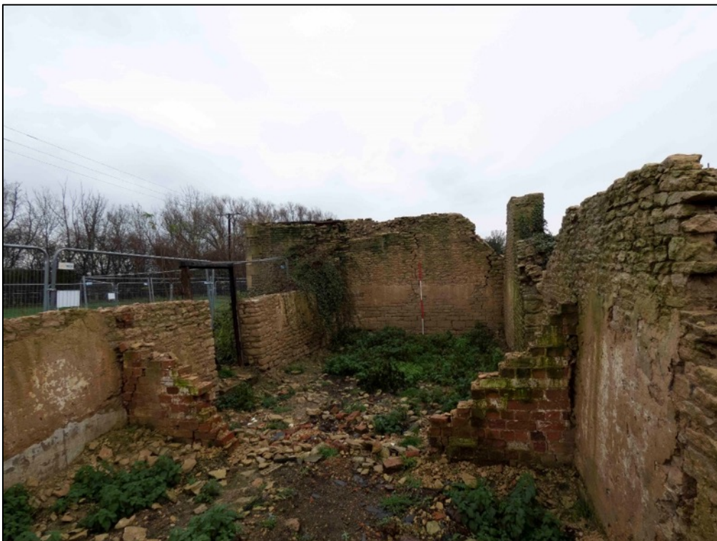
Appendix 2.54 View of rooms 2G1-2G2, Barn 2, looking north-west (2018)
