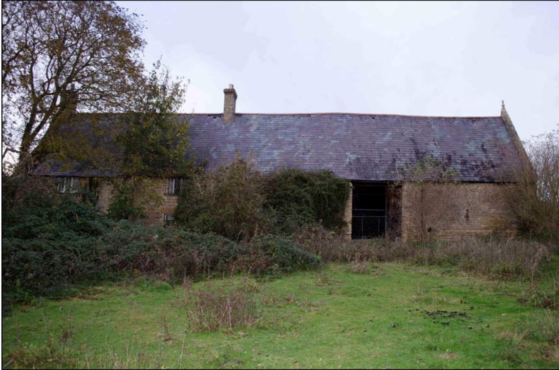
Appendix 2.9 View of Cottages 1 & 2 and Barn 1, looking north-west (2018)
