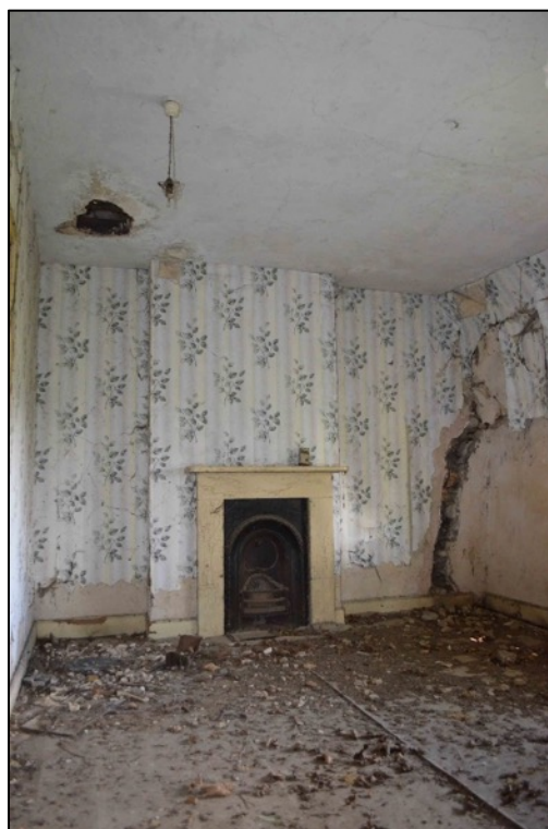
Appendix 2.18 View of room IF6, Cottage I, looking north-east (2019)
