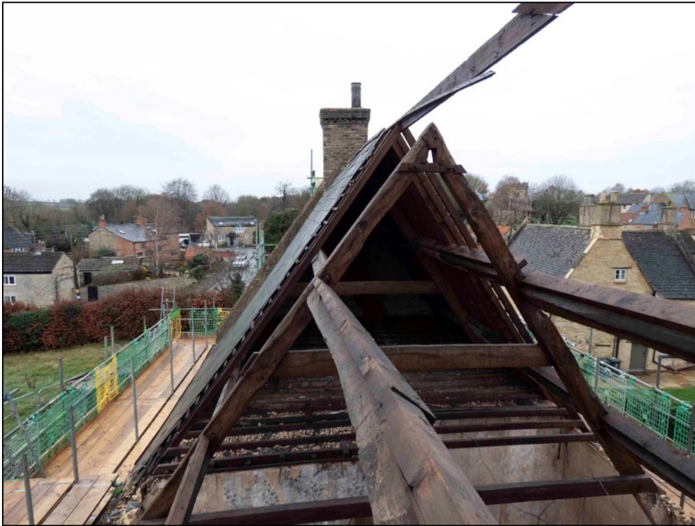
Appendix 2.35 Detail of truss above Cottage I , looking south-east
