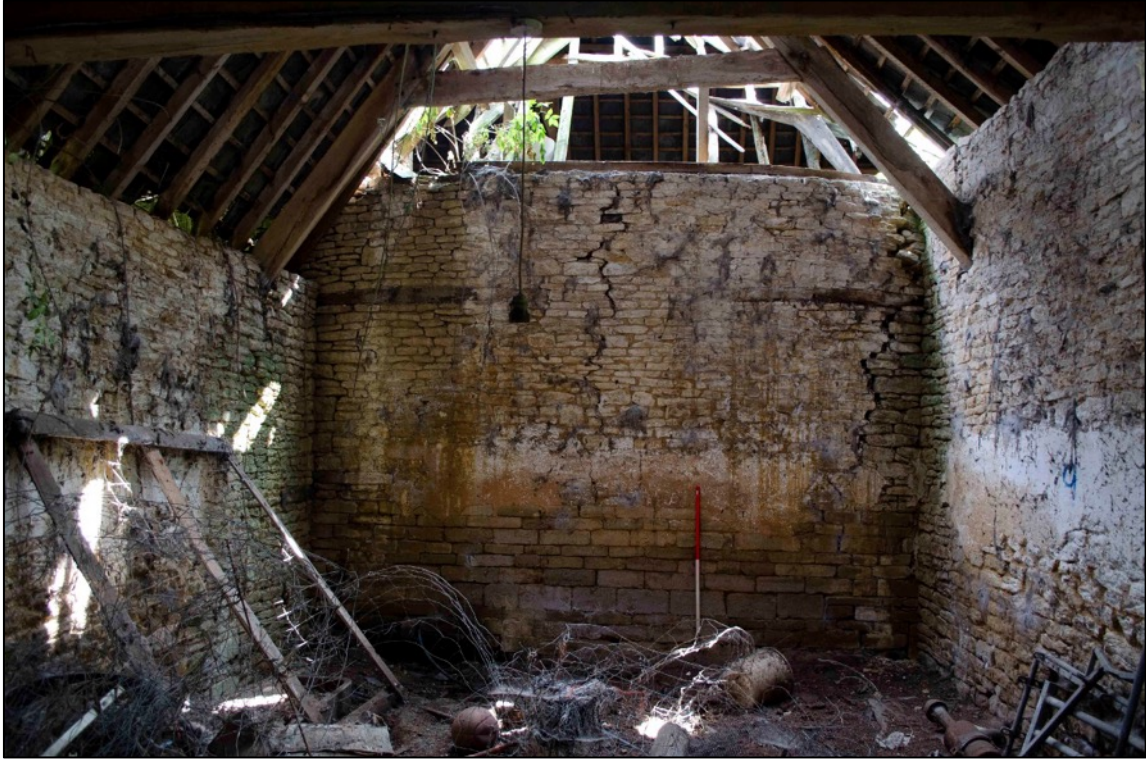
Appendix 2.51 View of room 2G1, Barn 2, looking south-east (2018)
