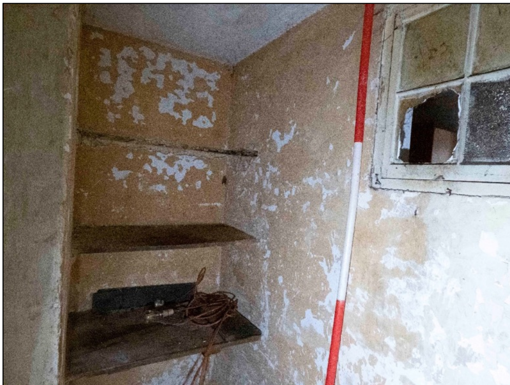
Appendix 2.26 View of room IG4 Cottage 2, looking west (2023)
