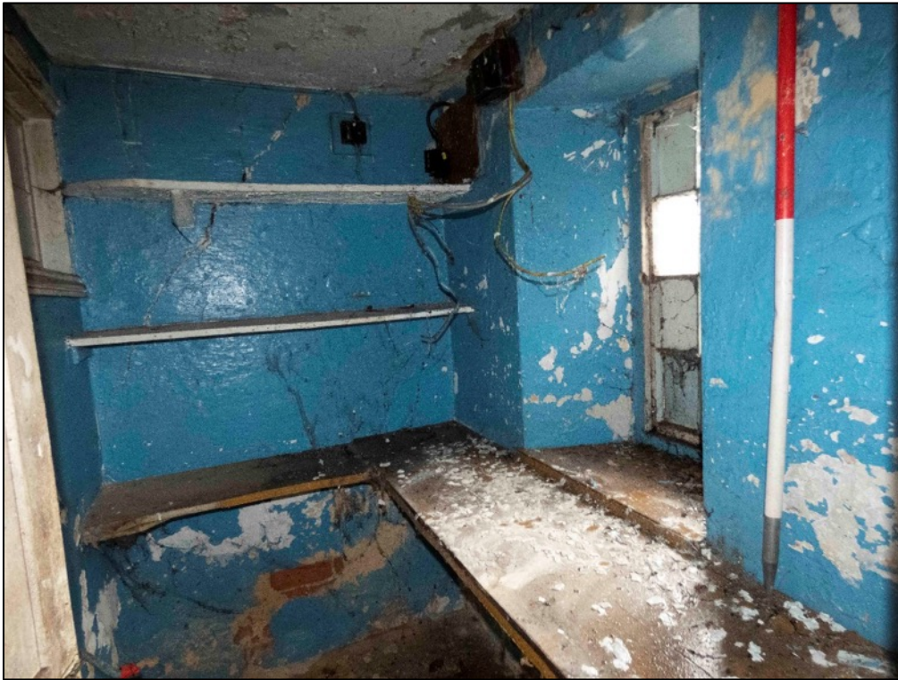
Appendix 2.17 View of room IG7, Cottage I, looking west (2023)
