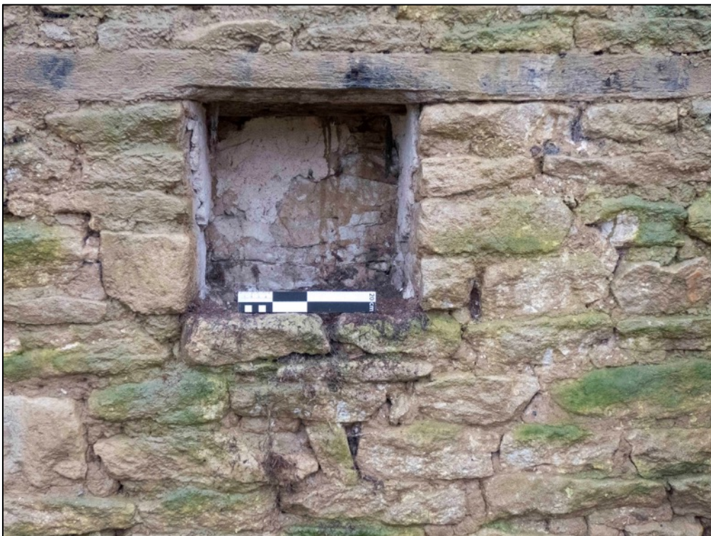
Appendix 2.56 Detail of niche in south-west wall of room 2G1, Barn 2 (2023)
