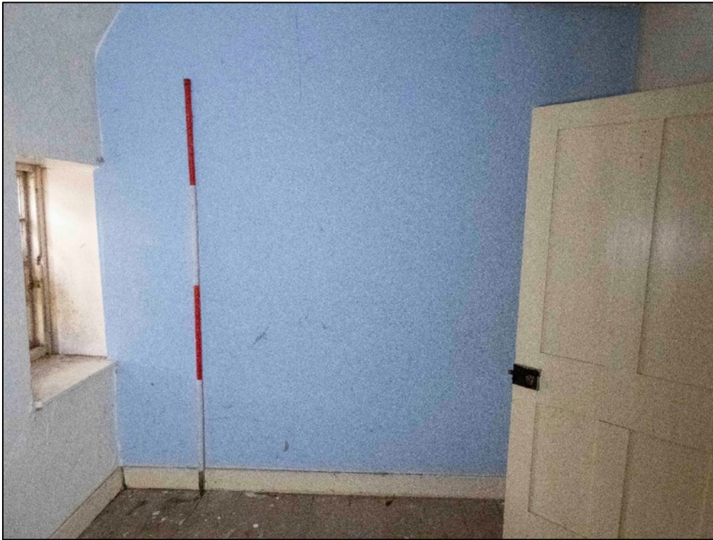
Appendix 2.29 View of room IF4 Cottage 2, looking north-east (2023)
