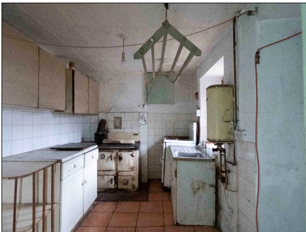
Appendix 2.22 View of room IG2 Cottage 2, looking south-west (2023)
