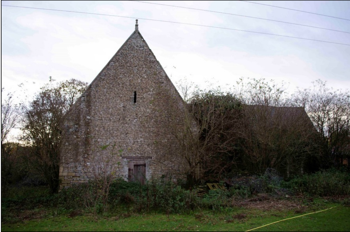
Appendix 2.37 North-east gable of Barn I , looking south-east (2018)
