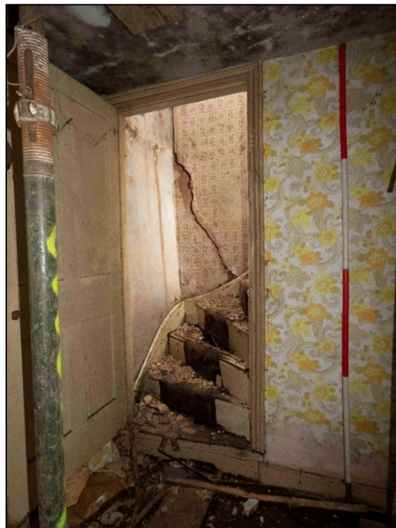
Appendix 2.16 Detail of stairs in room IG5, Cottage I, looking south-west (2023)
