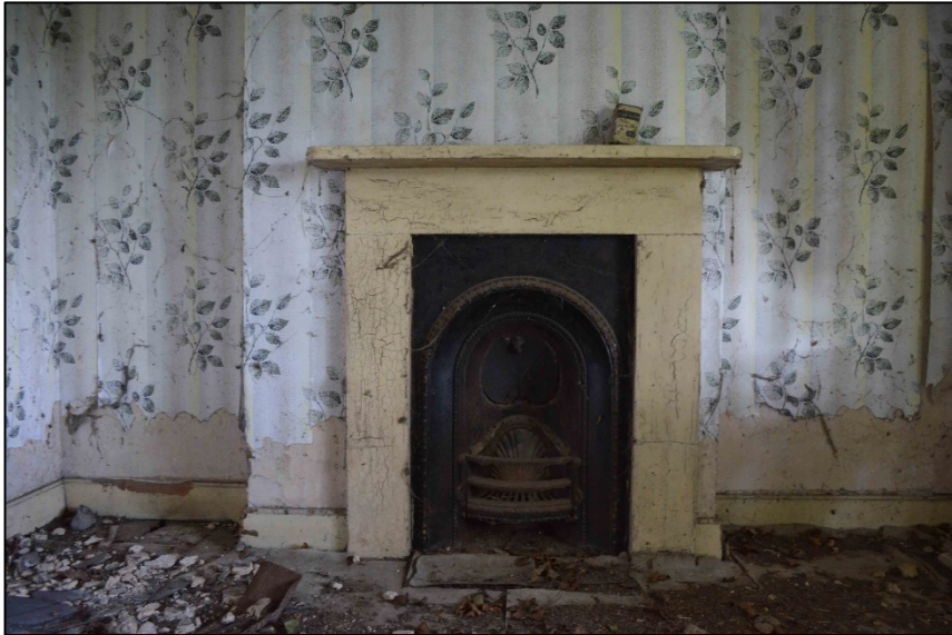
Appendix I.10: Detail of fireplace in room IF6, Cottage 1 , looking north-east (2019)
