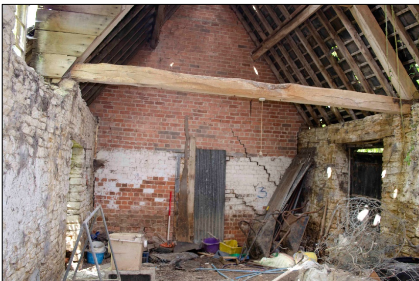
Appendix I.18: View of room 2G1 of the Barn , looking north-west (2018)
