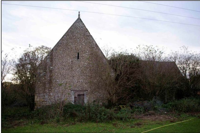
Appendix 1.13: North-east gable of Barn , looking south-east (2018)
