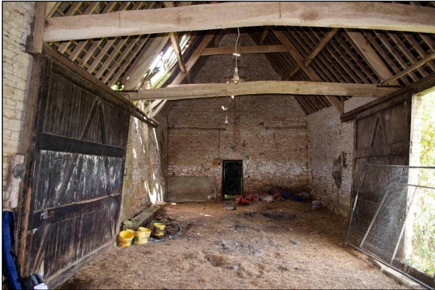
Appendix I.16: View of room IG9 of the Barn , looking north-east (2018)
