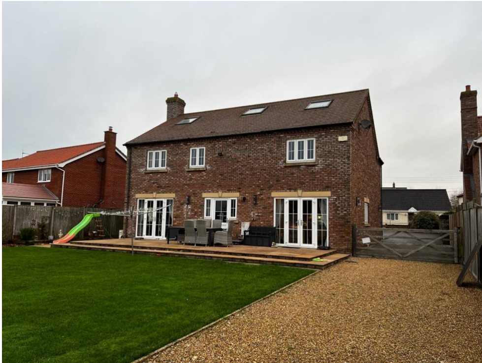
Photograph showing existing rear of Fieldview.
