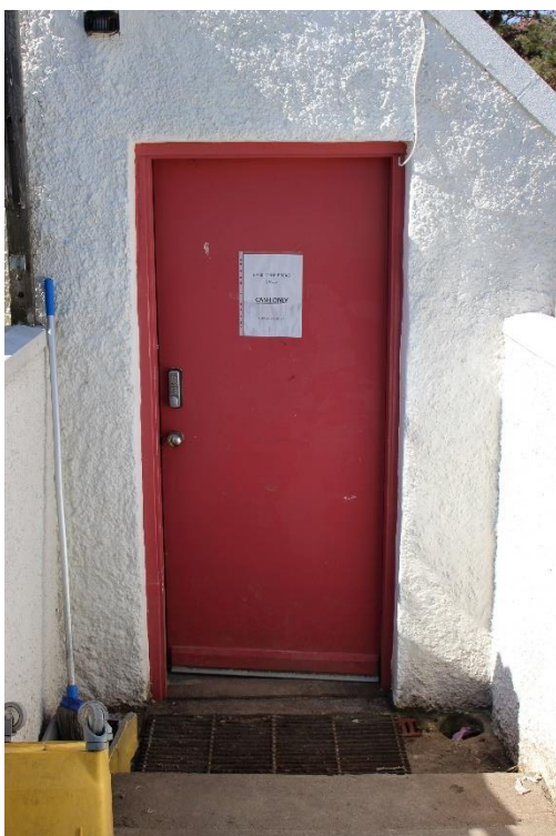
2. Existing rear door
