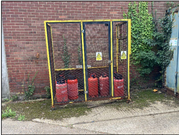
Plate 7. Gas tank container cage on northern perimeter of Site.
