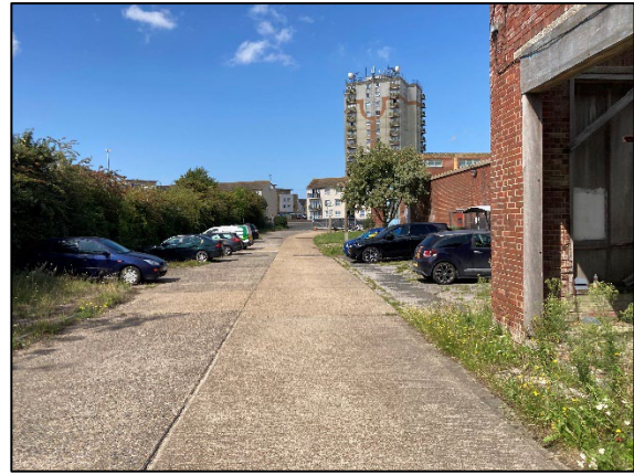
Plate 2. View of parking along factory perimeter.
