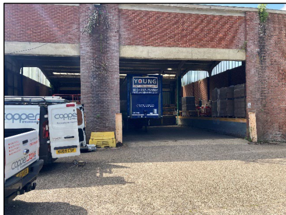
Plate 15. View of factory loading bay.
