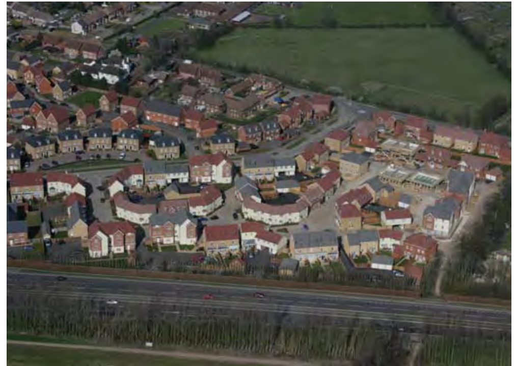
SCOTT AVENUE, CANTERBURY
