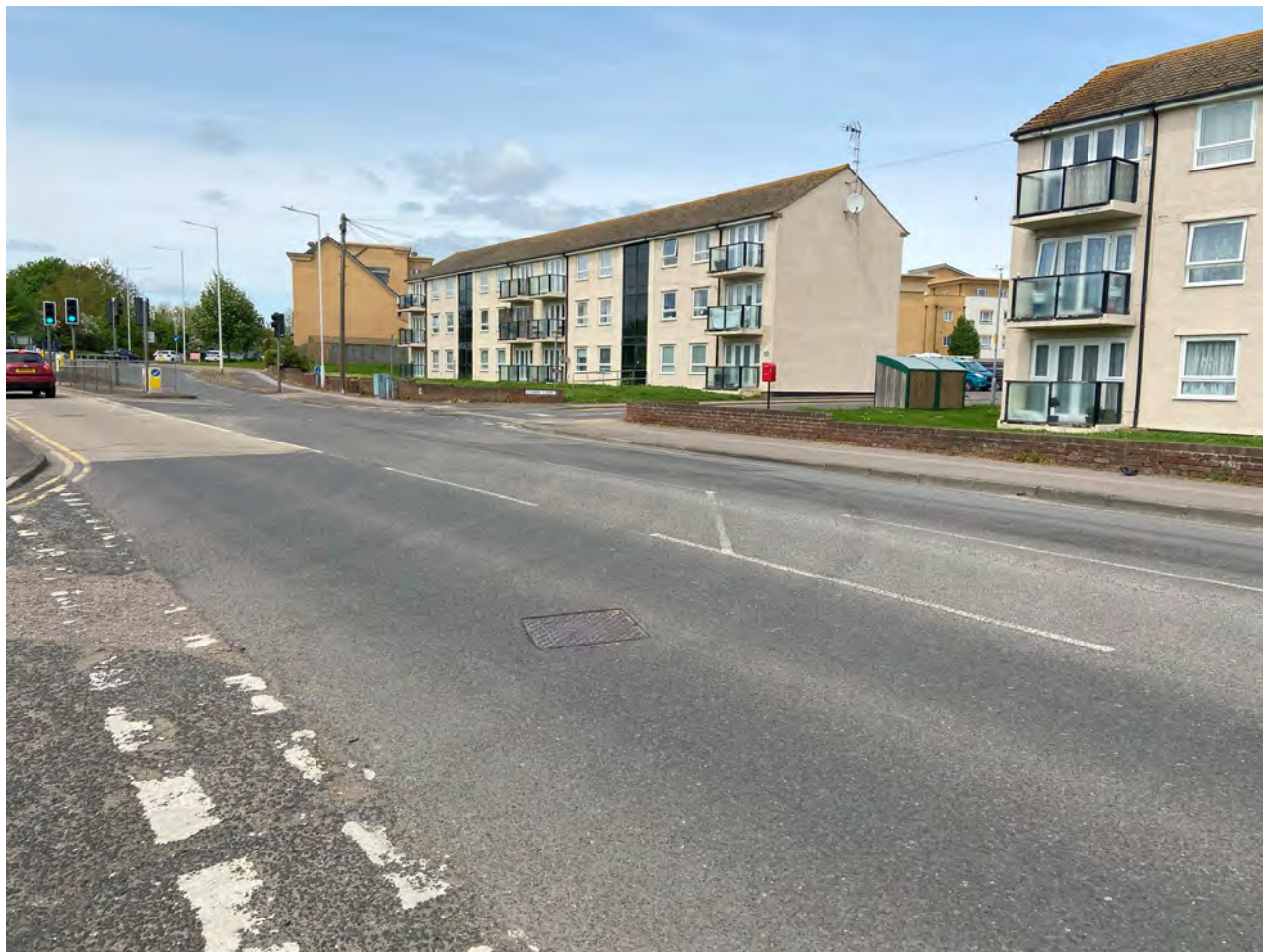
Photograph 3.2: Manston Road in a North West Direction from the Site Entrance
