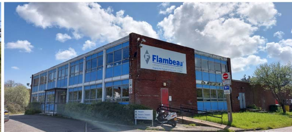
Northern and western elevations of B1
