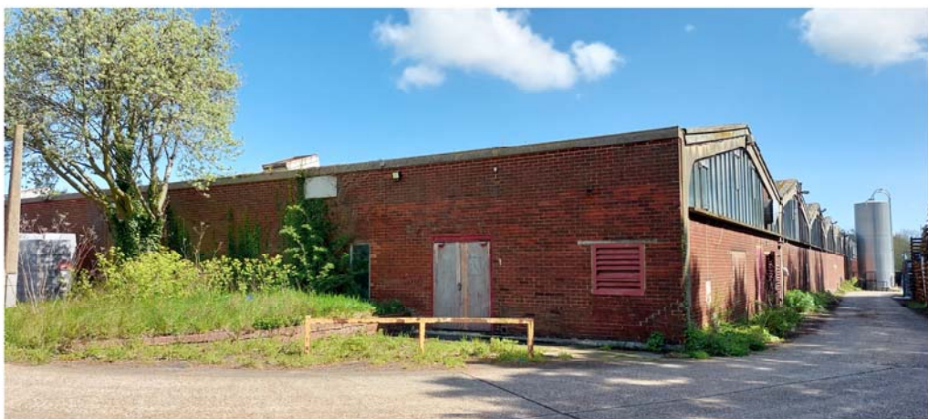
Western and southern elevations of B1
