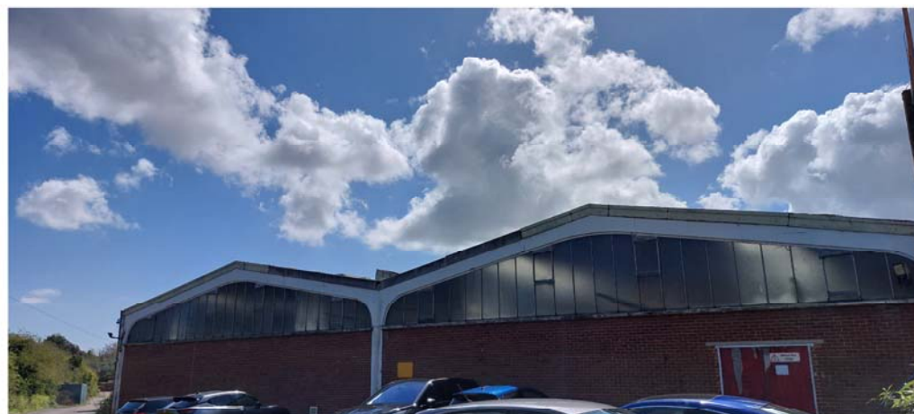
Northern elevation of B1
