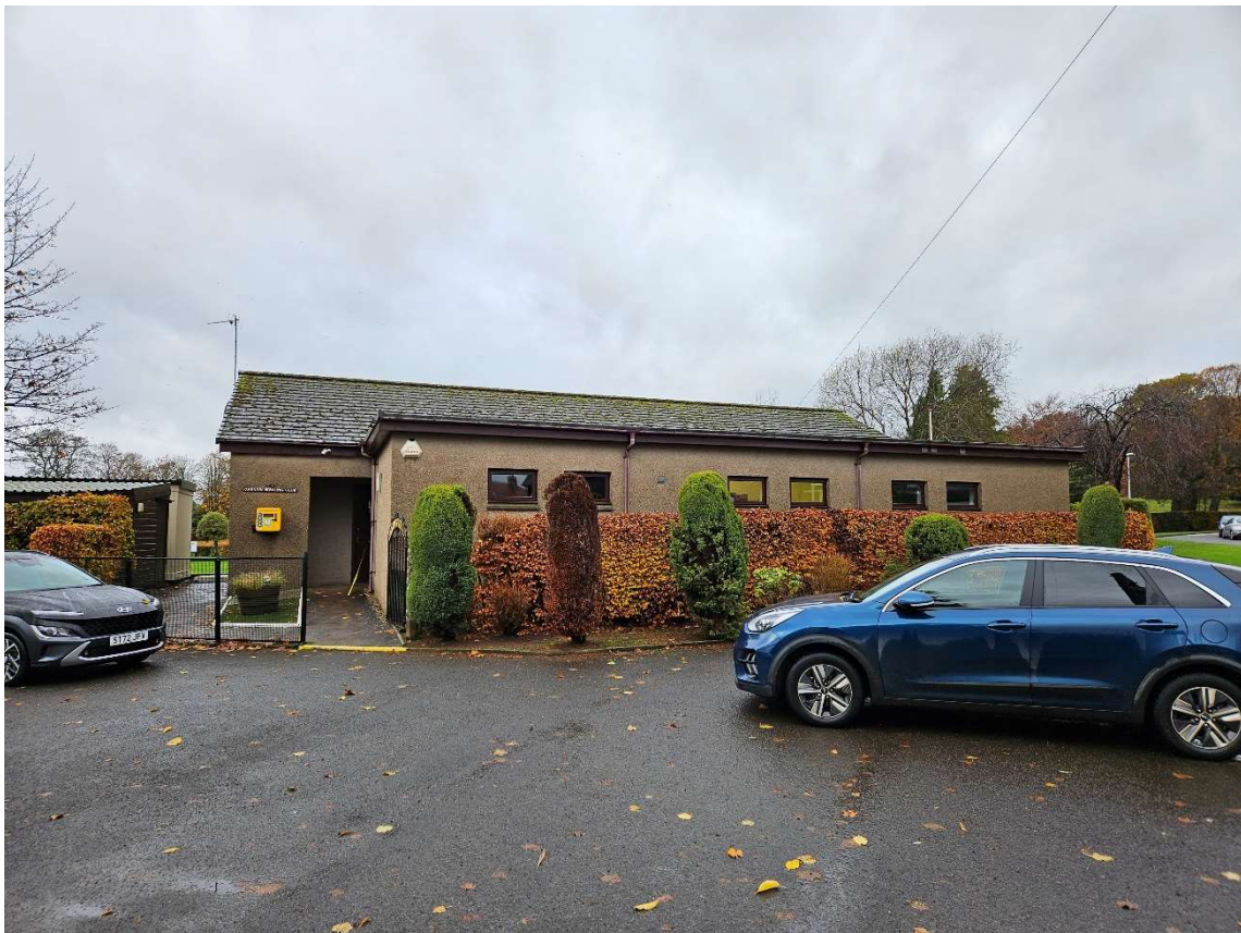
View of the East Elevation from the Car Park
