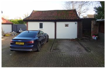
The single storey office building comprising of clay lump walls on brick and flint quoined plinths under a pitched pantile roof with painted timber joinery.
