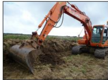
PHOTOGRAPH 4 - EXPOSING OF TIMBERS ON SOUTH FACE
