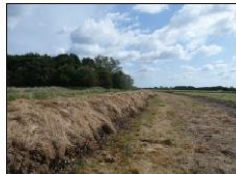
PHOTOGRAPH 6 - COMPLETED HIBERNACULA BANK
