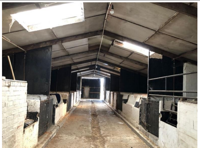
Photo 12 The interior of the existing building
