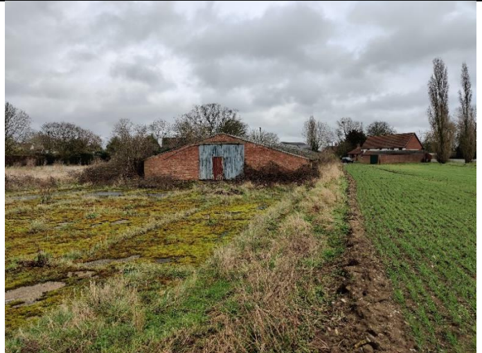
Photo 2 The western elevation of the building, with tall vegetation, scrub and the arable field to the south.
