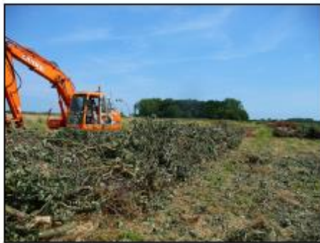
PHOTOGRAPH 3 - BRASH PLACED OVER REED BUNDLES AND LARGE TIMBERS
