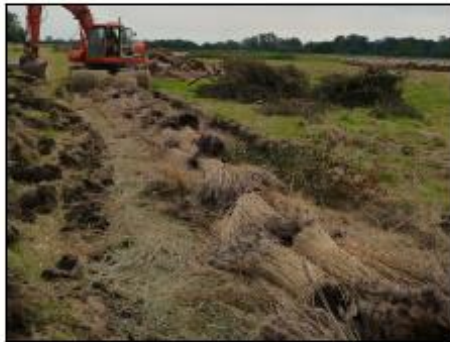
PHOTOGRAPH 1 - CENTRAL CORE PLACED OF REED BUNDLES AND RUSH BALES
